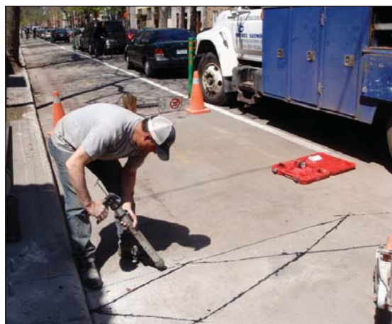
Exhibit 17: Installing a permanent cyclist counting station in Montreal, QC
