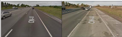
Trial section location before (left) and after (right) construction (Google Maps, 2015 & 2016)
