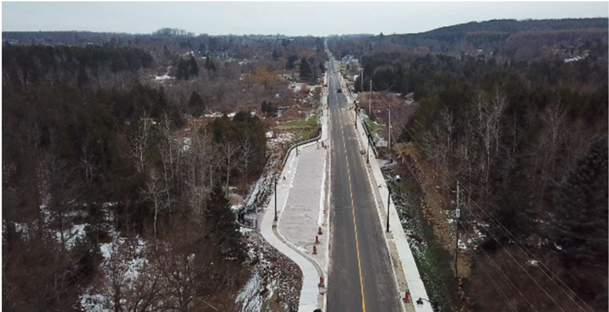
Figure 3-4: Parking Lay-By at Queen Street East
