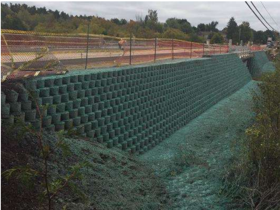
Figure 3-7 – Vegetated Retained Soil Slopes
