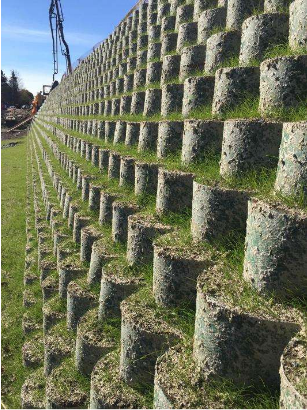
Figure 3-7 – Vegetated Retained Soil Slopes
