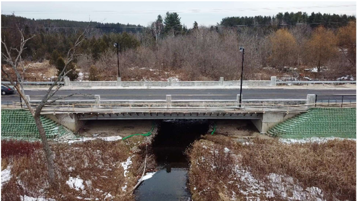
Figure 3-10 – Shaw's Creek Bridge
