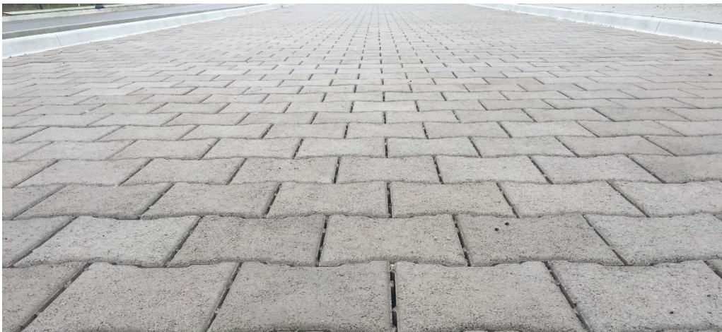
Figure 3-5: Permeable Pavement at Parking Lay-By at Queen Street East
