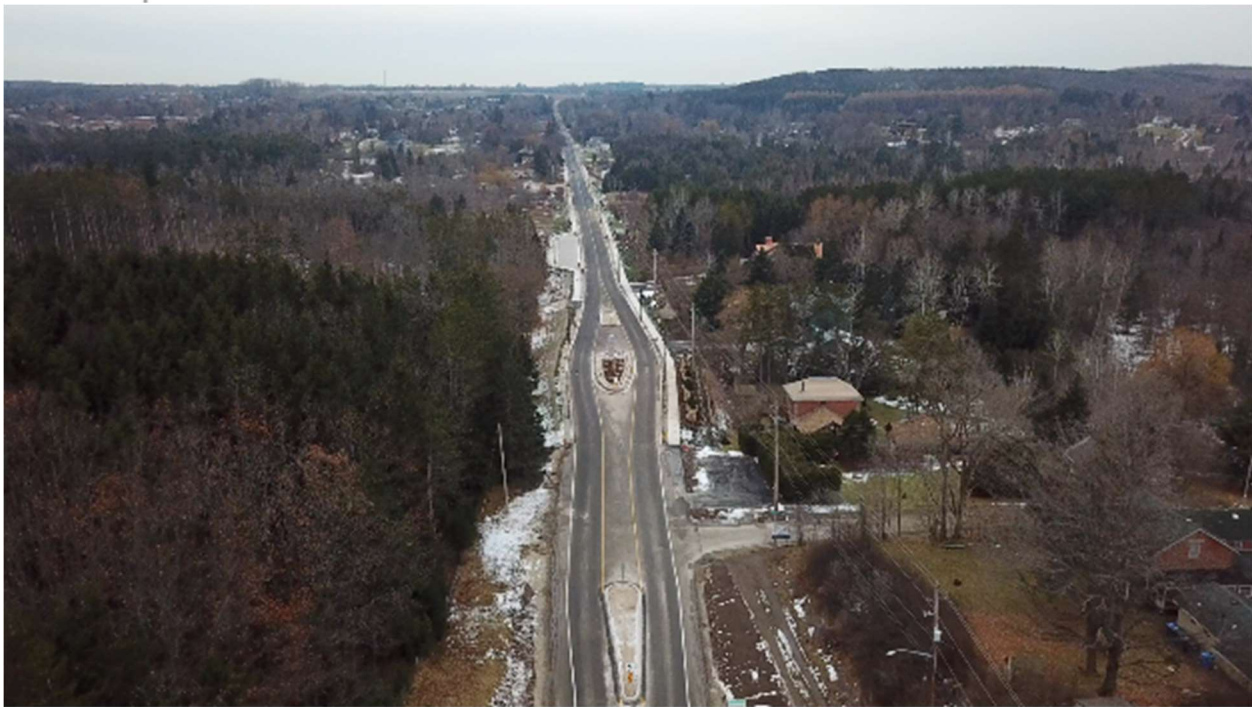
Figure 3-2: Traffic Calming Islands at Queen Street East
