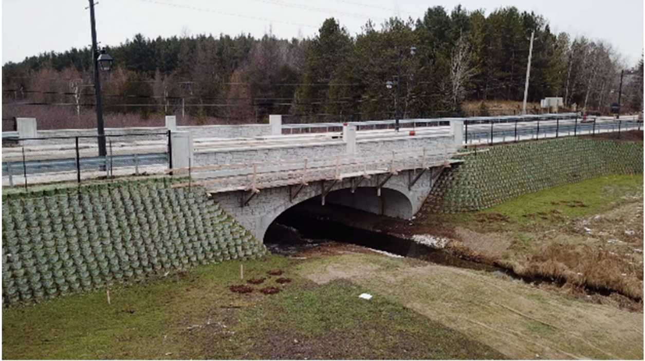
Figure 3-11 – Culvert Bridge at Shaw’s Creek Tributary
