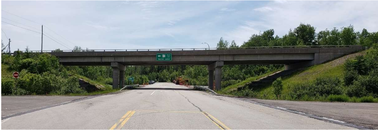
Figure 1: W475 Westfield overpass.
