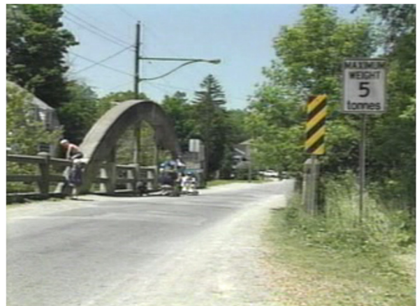
1994 Video with unsafe behaviours at the side of the bridge
