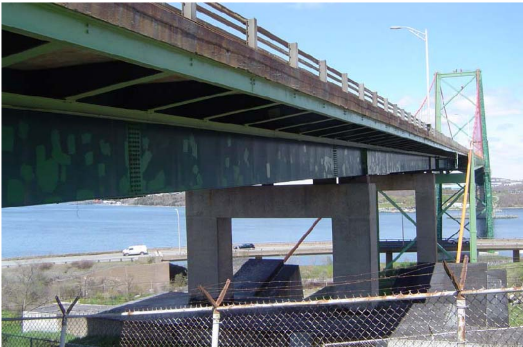
Figure 2. Halifax Approach Span (courtesy B&T)
