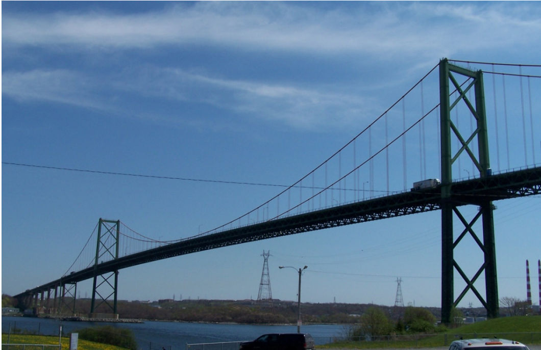
Figure 1. A Murray MacKay Bridge
