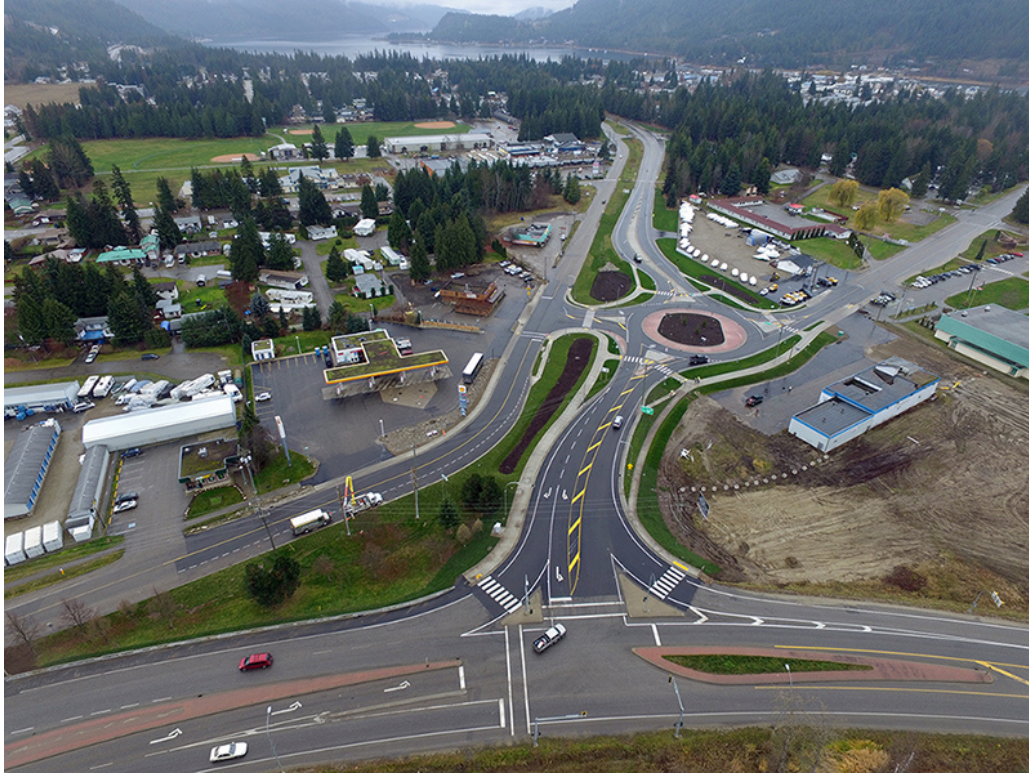
Figure 9 – Roundabout as constructed
