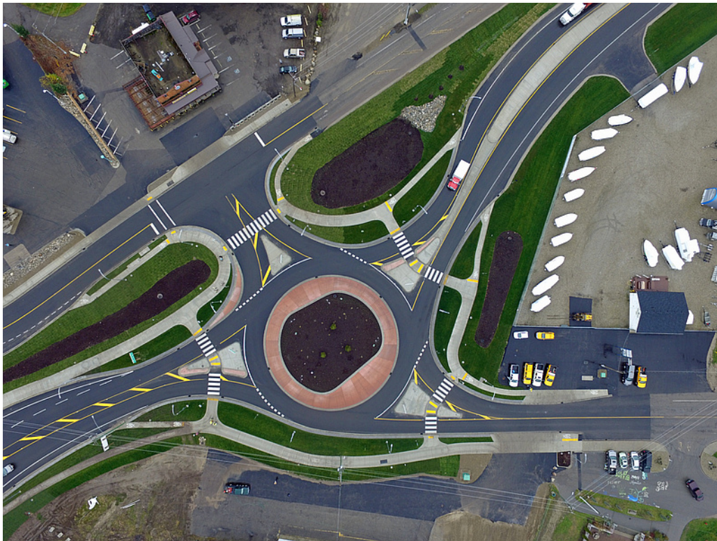
Figure 10 – Roundabout as constructed
