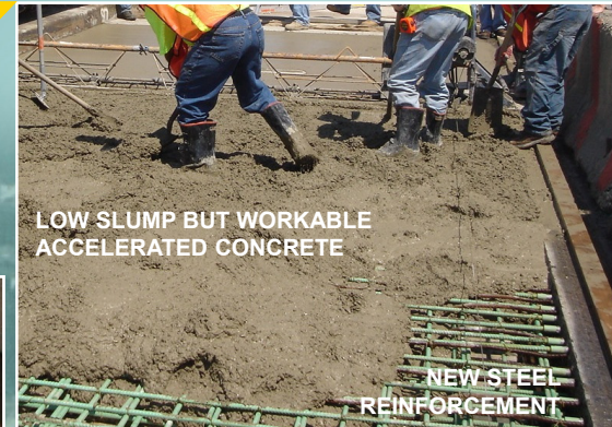
RECONSTRUCTION OF TEST SPAN
