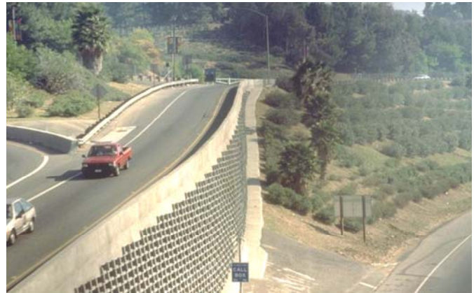
Figure 7 Damage to Road Shoulder on an On-Ramp to Highway 101, Universal City, LA, USA (1994 Northridge Earthquake)
