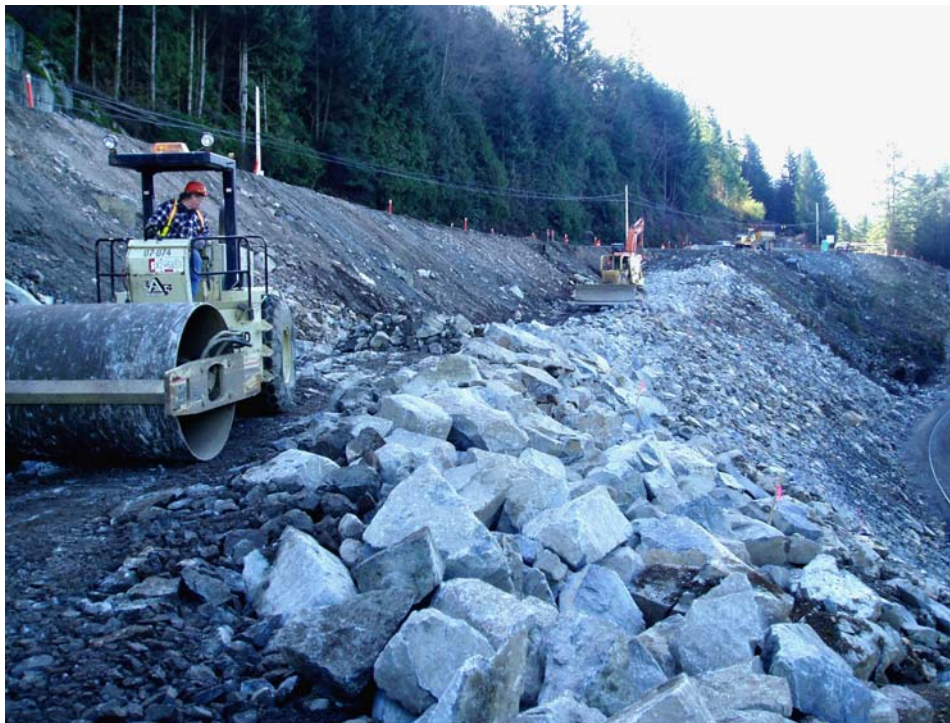
Figure 8 Construction of Rock Fill Slope to Support MSE Retaining Wall
