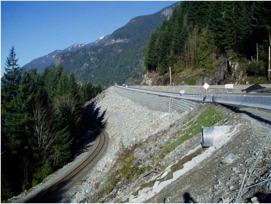
Figure 9 Completed MSE Retaining Wall on Rock Fill Slope
