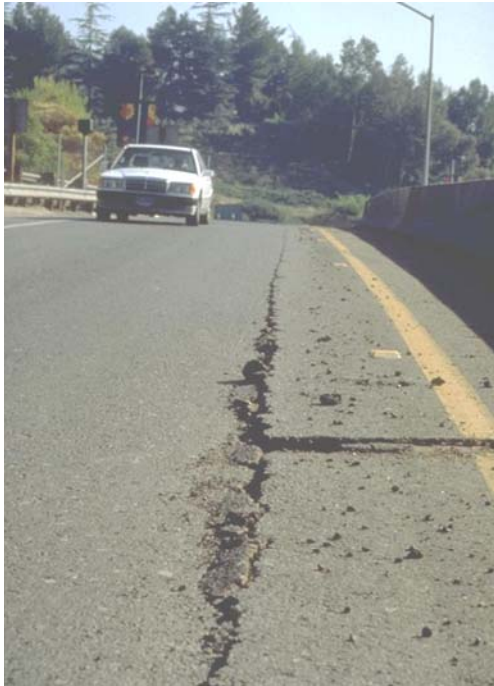
Figure 7 Damage to Road Shoulder on an On-Ramp to Highway 101, Universal City, LA, USA (1994 Northridge Earthquake)
