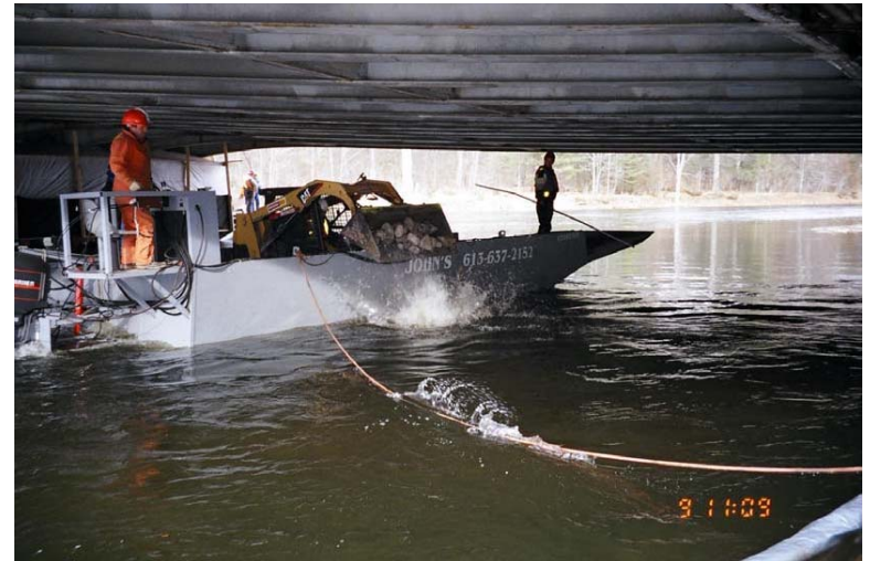
Figure 7: Installing rock liner under structure. Photo
