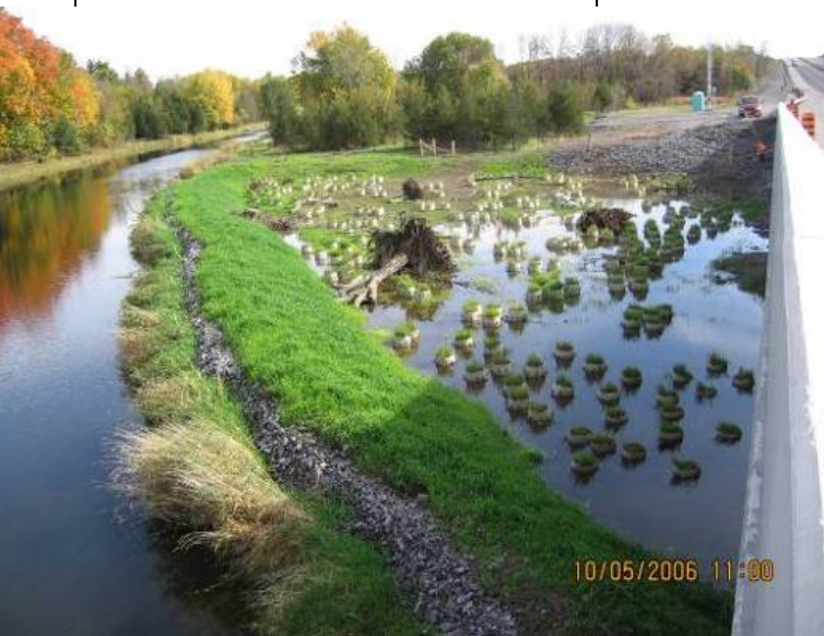
Figure 6: NW quadrant of Bridge. Completed pike spawning habitat design. Photo by Jewel Eng.
