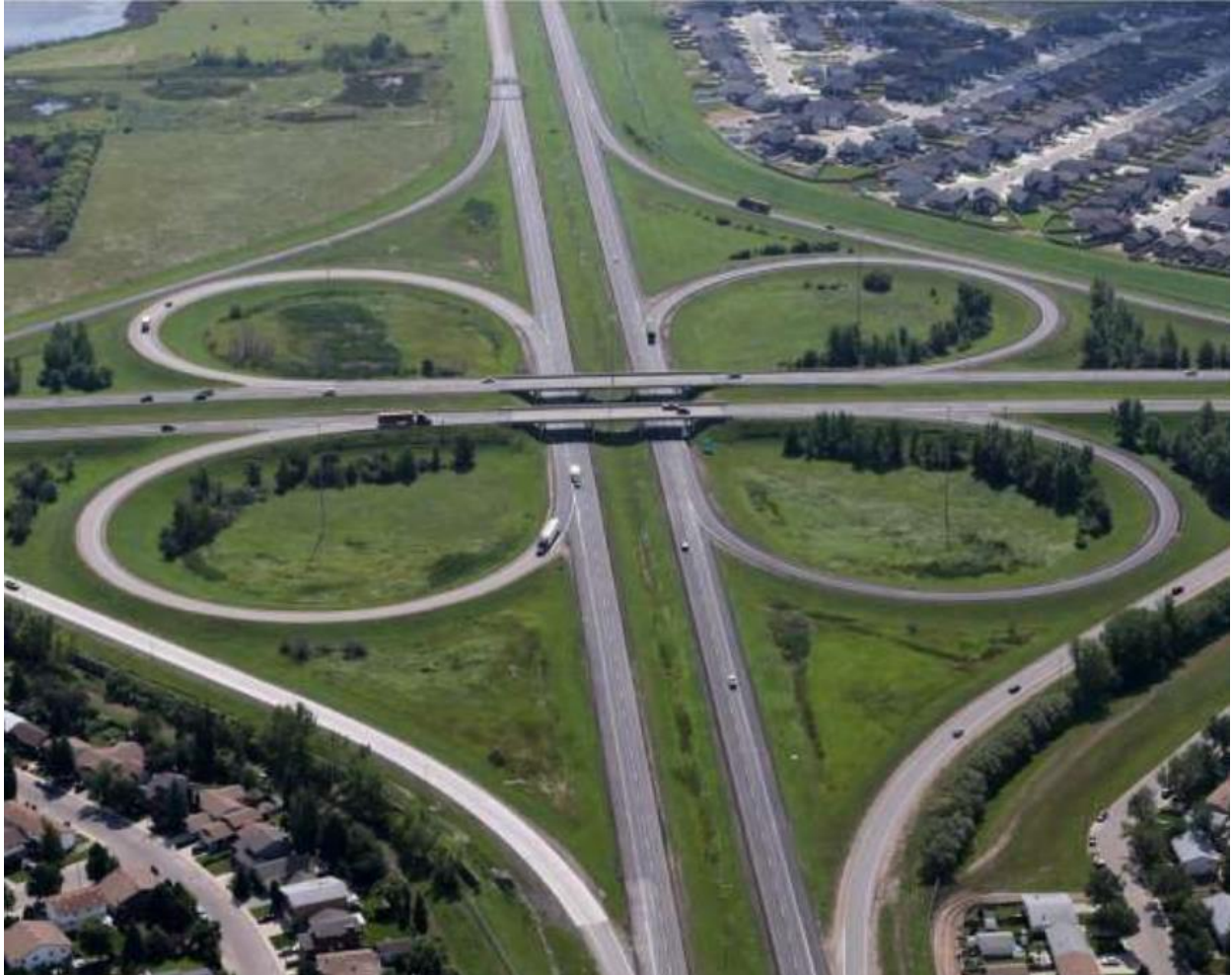
Figure 2: Existing Cloverleaf Interchange, Looking South
