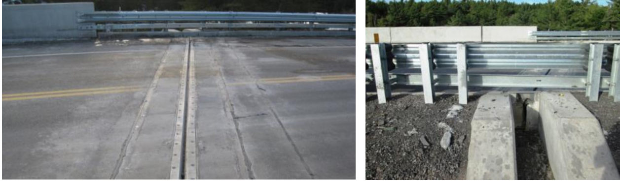
Fig. 14: Expansion joint at the end of an approach slab
