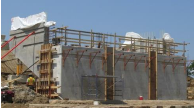
Fig. 17: Two approaches to prefabricated abutments: (a) precast concrete components emulating a cast-in-place abutment and (b) example of semi-integral abutment with girders supported on pier cap on piles and earth retained by separate sheet pile retaining wall system
