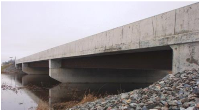
Fig. 12: Steel girder bridge with integral abutments and integral piers
