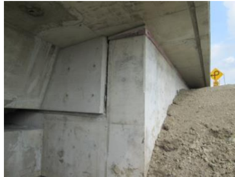
Fig. 11: Semi-integral abutment details with barrier continuous from the deck onto the approach slab which overhangs beyond the wingwall
