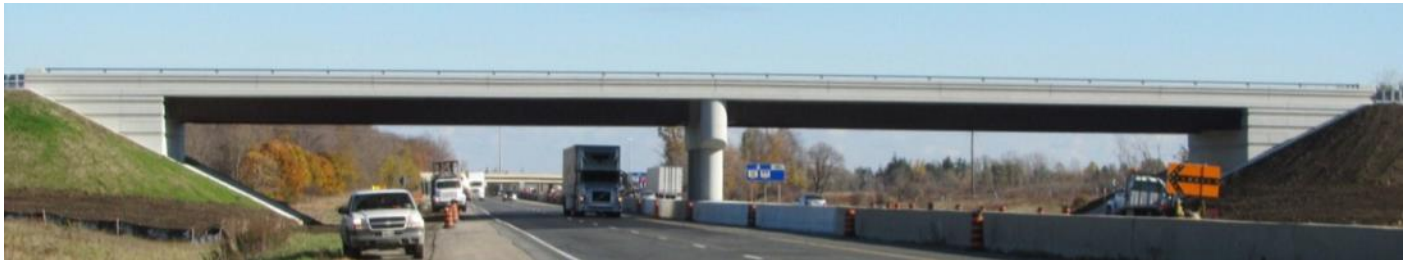
Fig. 16: Westminster Drive Underpass over Hwy 401
