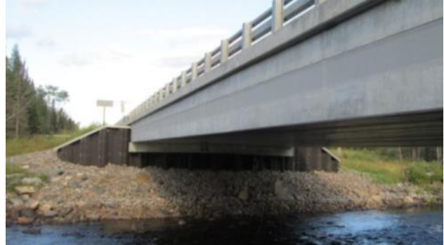
Fig. 17: Two approaches to prefabricated abutments: (a) precast concrete components emulating a cast-in-place abutment and (b) example of semi-integral abutment with girders supported on pier cap on piles and earth retained by separate sheet pile retaining wall system
