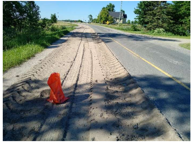
3 Figure 3 Partly pulverized pavement sections (left: Niagara-on-the-Lake, right: Bruce 4 County)
