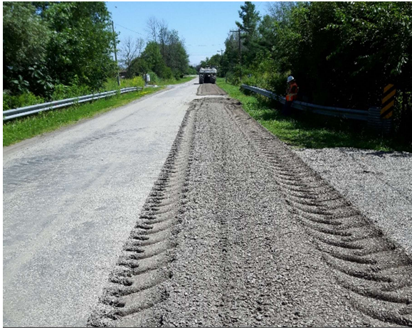
3 Figure 3 Partly pulverized pavement sections (left: Niagara-on-the-Lake, right: Bruce 4 County)
