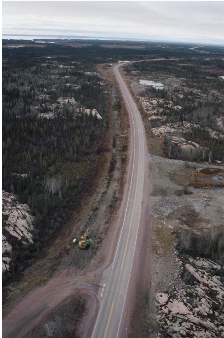
Figure 2 - Yellowknife Highway After Reconstruction
