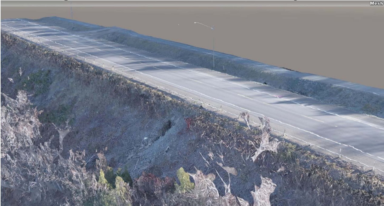
Figure 4: UAV Mesh Model of Route 105 embankment facing North
