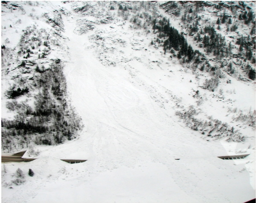
FIGURE 2 Avalanche over Snowshed (Photo Courtesy of Parks Canada)
