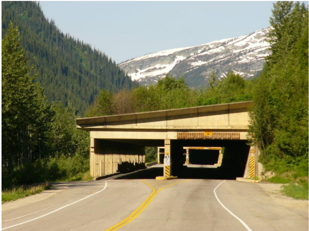
FIGURE 1 Avalanche Snow Shed (photo courtesy of Parks Canada)
