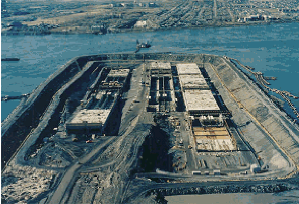
FIGURE 5 Casting Basin for Pre-stressed segments Lafontaine Tunnel (5)
