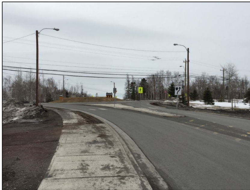
Figure 16 - Hardy Avenue, Grenfell Heights and Scott Avenue Roundabout in Grand Falls- Windsor, NL
