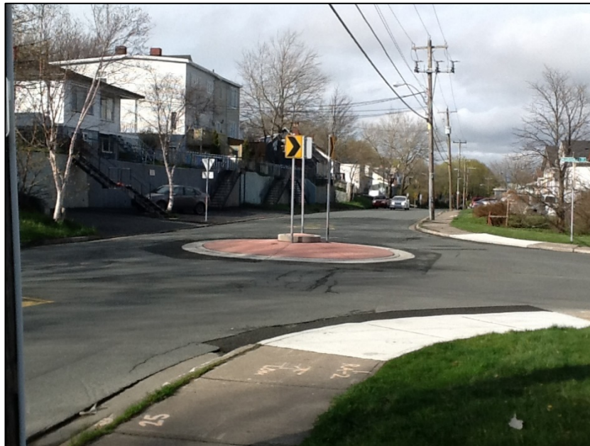
Figure 7 - Traffic circle on Old Topsail Road
