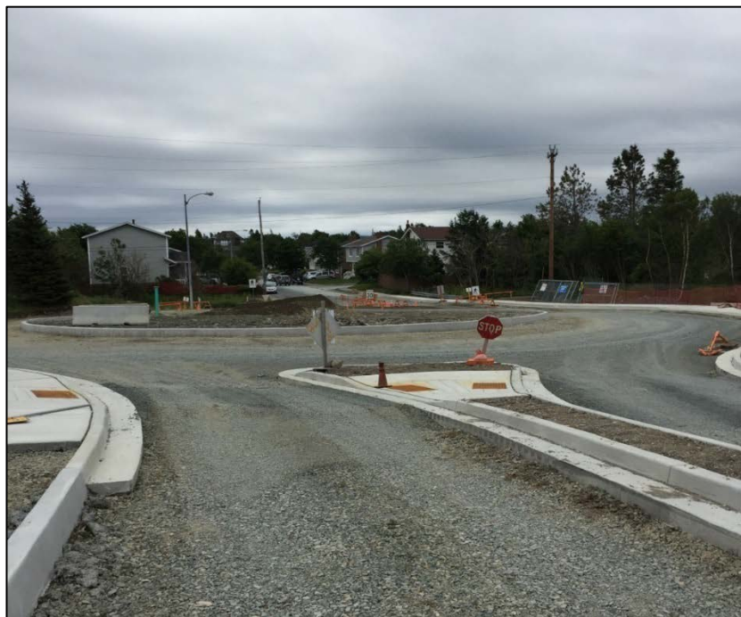
Figure 15 - Carrick Drive Roundabout at the Paul Reynolds Community Centre [16]
