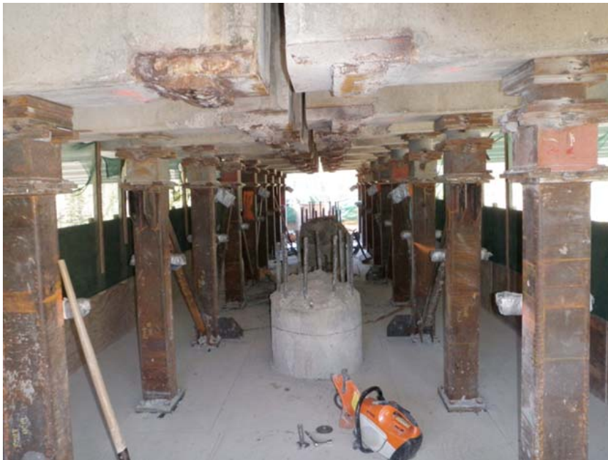
Figure 10) Support system beneath jacked girders during reconstruction of pier cap
