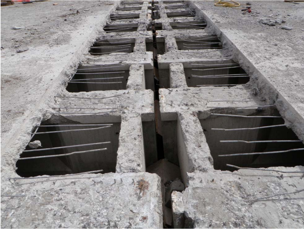
Figure 12) Link slab after chipping away of existing deck
