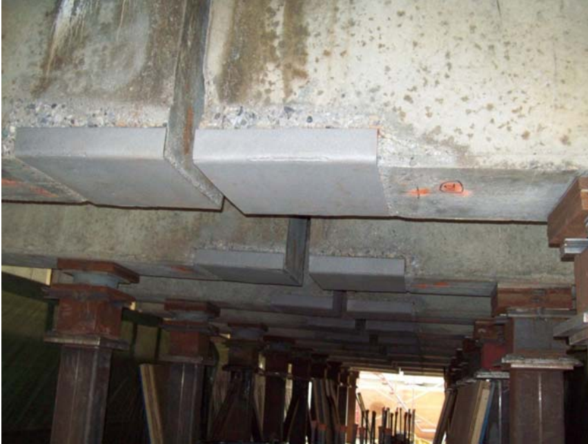
Figure 11) Existing sole plates sandblasted and metalized for use with new bearings
