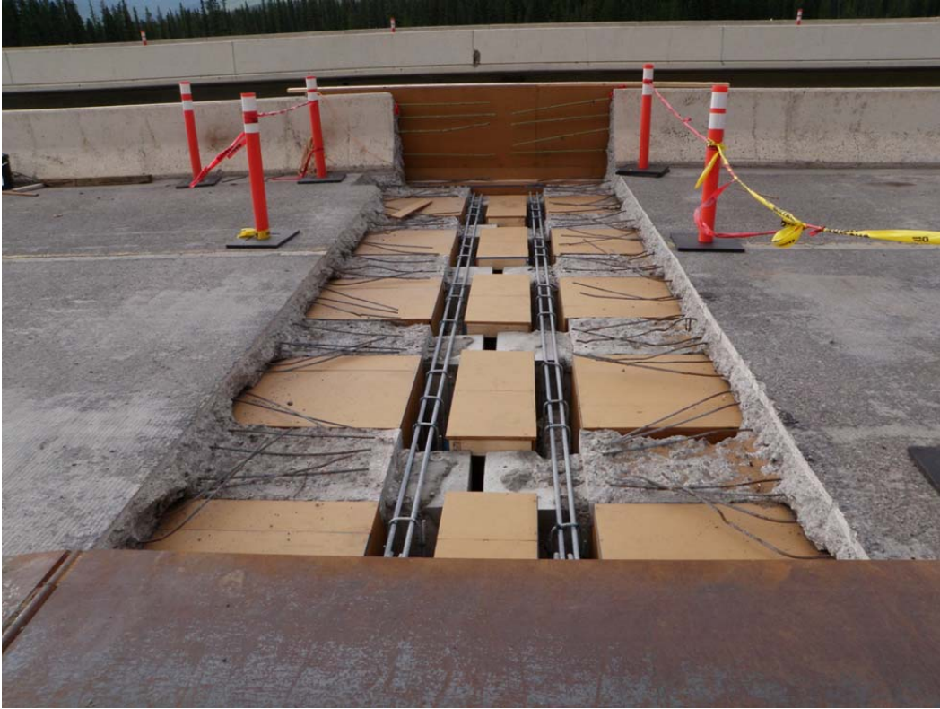
Figure 13) Formwork in place for the concrete diaphragms and link slab deck
