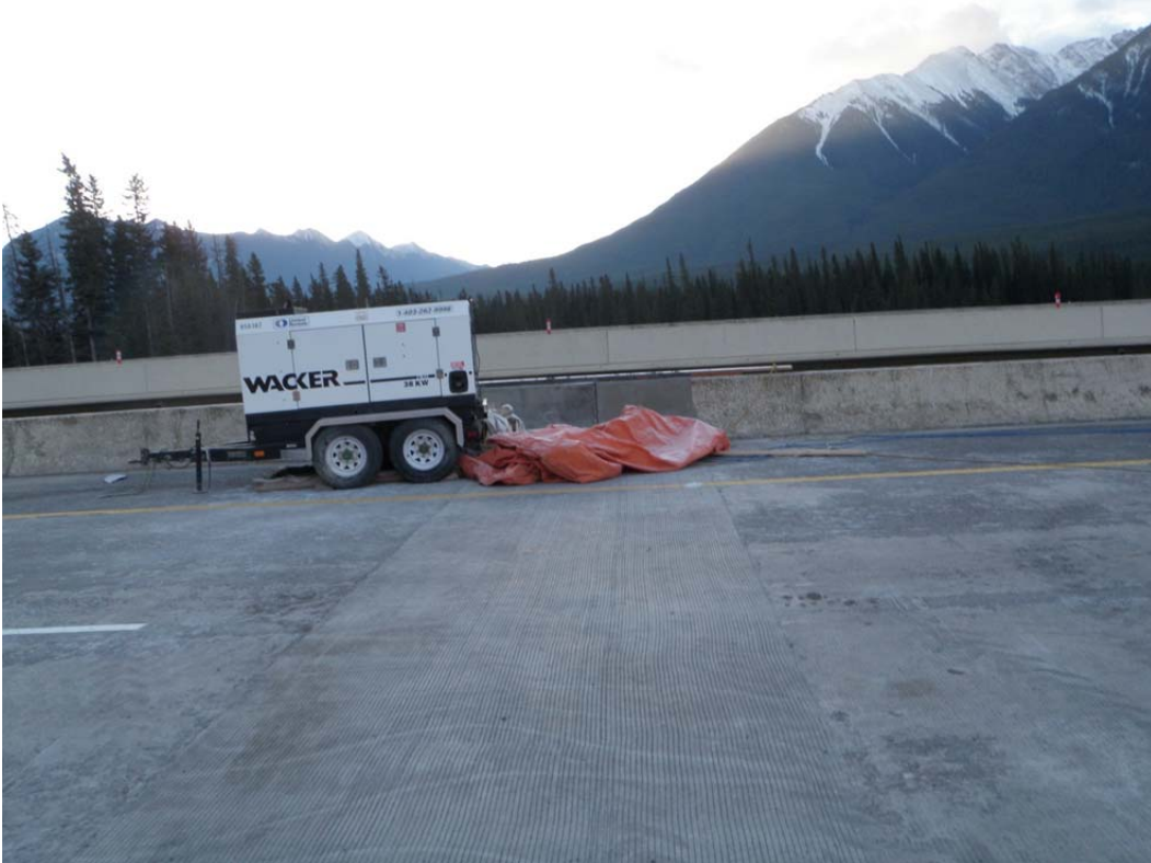
Figure 15) Finished link slab.
