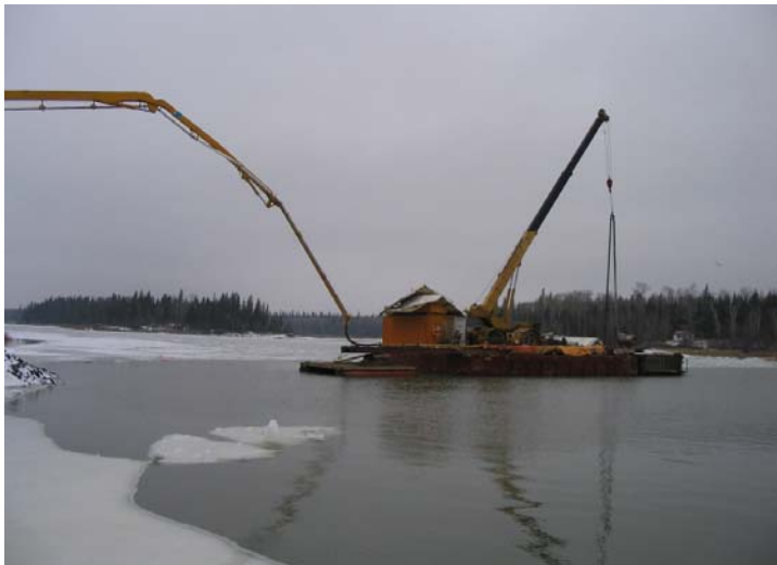
Photos 7 & 8: View of pumping and tremie placement operations for the river pier caissons.
