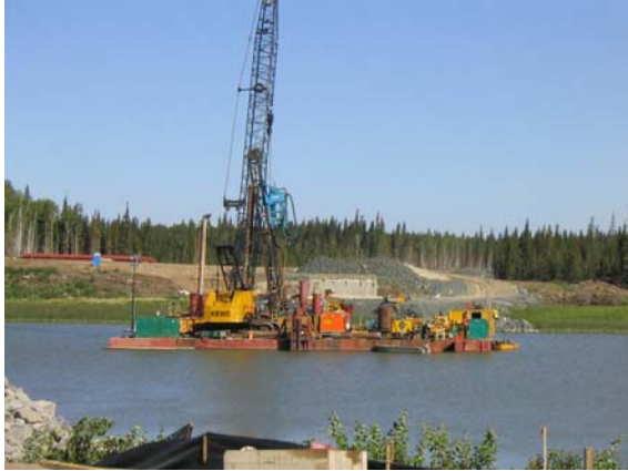
Photos 3 & 4: River pier foundations in the Nelson River constructed from barges utilizing a steel tub form.
