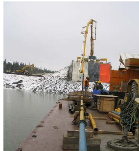
Photos 7 & 8: View of pumping and tremie placement operations for the river pier caissons.
