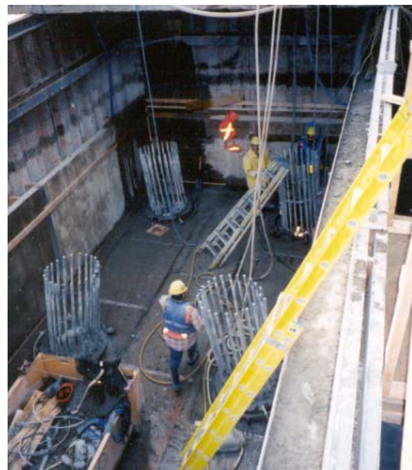
Photos 5 & 6: The steel tub form acted as both a template for the caisson installations, as well as a temporary cofferdam, which allowed construction of the underwater pile cap to be carried out in the dry.
