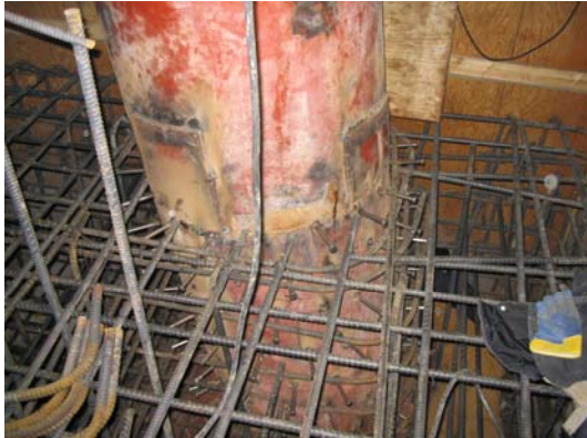
Photos 12 and 13: (Left) View of the steel Nelson studs welded onto the exterior of the sleeve as part of the modifications to provide fixity between the caisson and the pile cap. (Right) View of heated enclosure to facilitate coring, hydrodemolition and grouting operations, as well as dywidag installations off the ice in cold weather.
