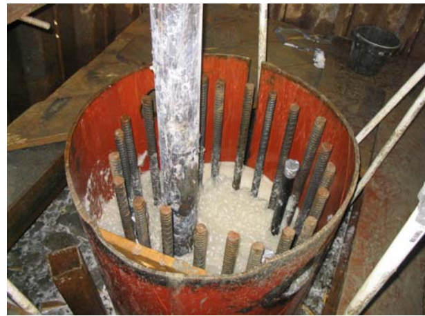
Photos 10 & 11: Close-up view of tremie placement at an individual caisson. Note the milky colour and foam in the water of the caisson that later required remediation.
