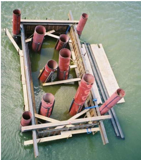
Photos 5 & 6: The steel tub form acted as both a template for the caisson installations, as well as a temporary cofferdam, which allowed construction of the underwater pile cap to be carried out in the dry.
