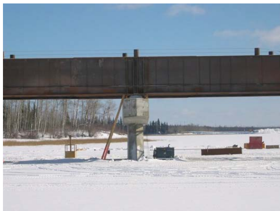
Photos 1 & 2: View of typical river piers illustrating the narrow, sloped pier shaft.
