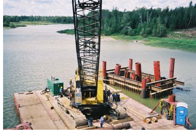
Photos 3 & 4: River pier foundations in the Nelson River constructed from barges utilizing a steel tub form.
