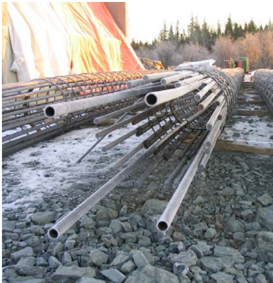
Photo 9 & Figure 4: Typical view of the caisson reinforcing cage illustrating the steel tubes for Crosshole Sonic Log (CSL) testing. Note the conduit layout facilitated two diagonal and four perimeter scans between the four tubes.
