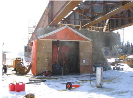
Photos 12 and 13: (Left) View of the steel Nelson studs welded onto the exterior of the sleeve as part of the modifications to provide fixity between the caisson and the pile cap. (Right) View of heated enclosure to facilitate coring, hydrodemolition and grouting operations, as well as dywidag installations off the ice in cold weather.
