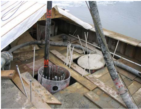
Photos 10 & 11: Close-up view of tremie placement at an individual caisson. Note the milky colour and foam in the water of the caisson that later required remediation.
