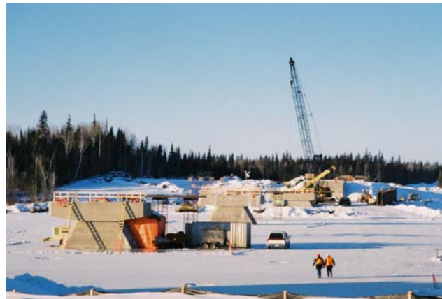
Photos 1 & 2: View of typical river piers illustrating the narrow, sloped pier shaft.
