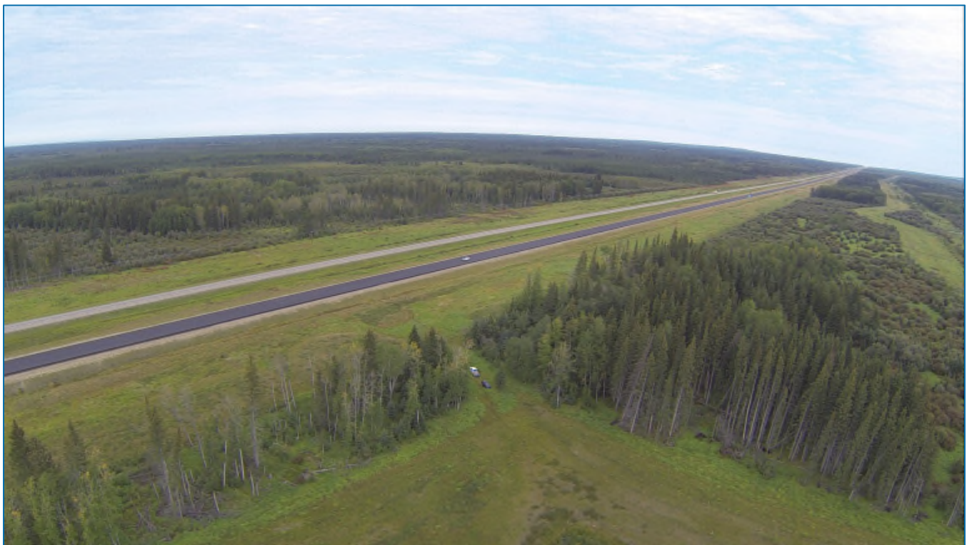
Figure 2: Aerial View of Newly Twinned Section of Highway 63
