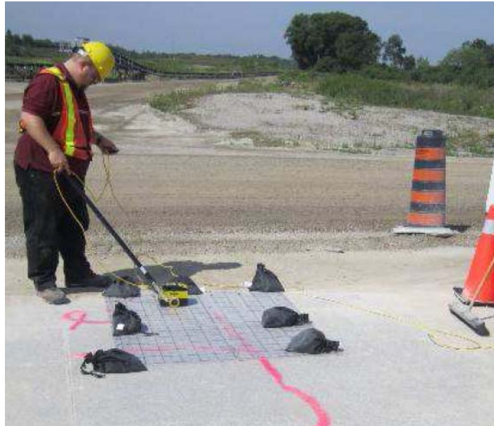
Figure 6: GPR being used to scan a 1200 x 1200 mm grid
