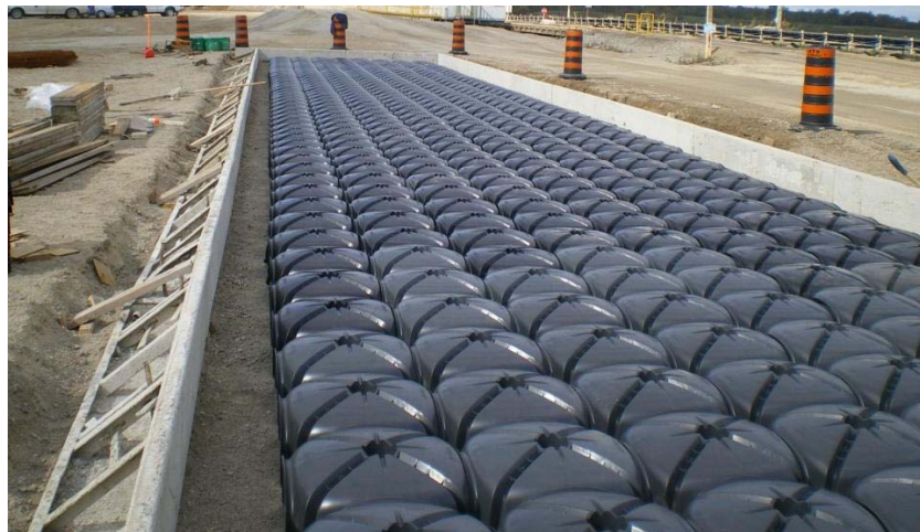
Figure 5: Typical Experimental Set Up of Cupolex System
