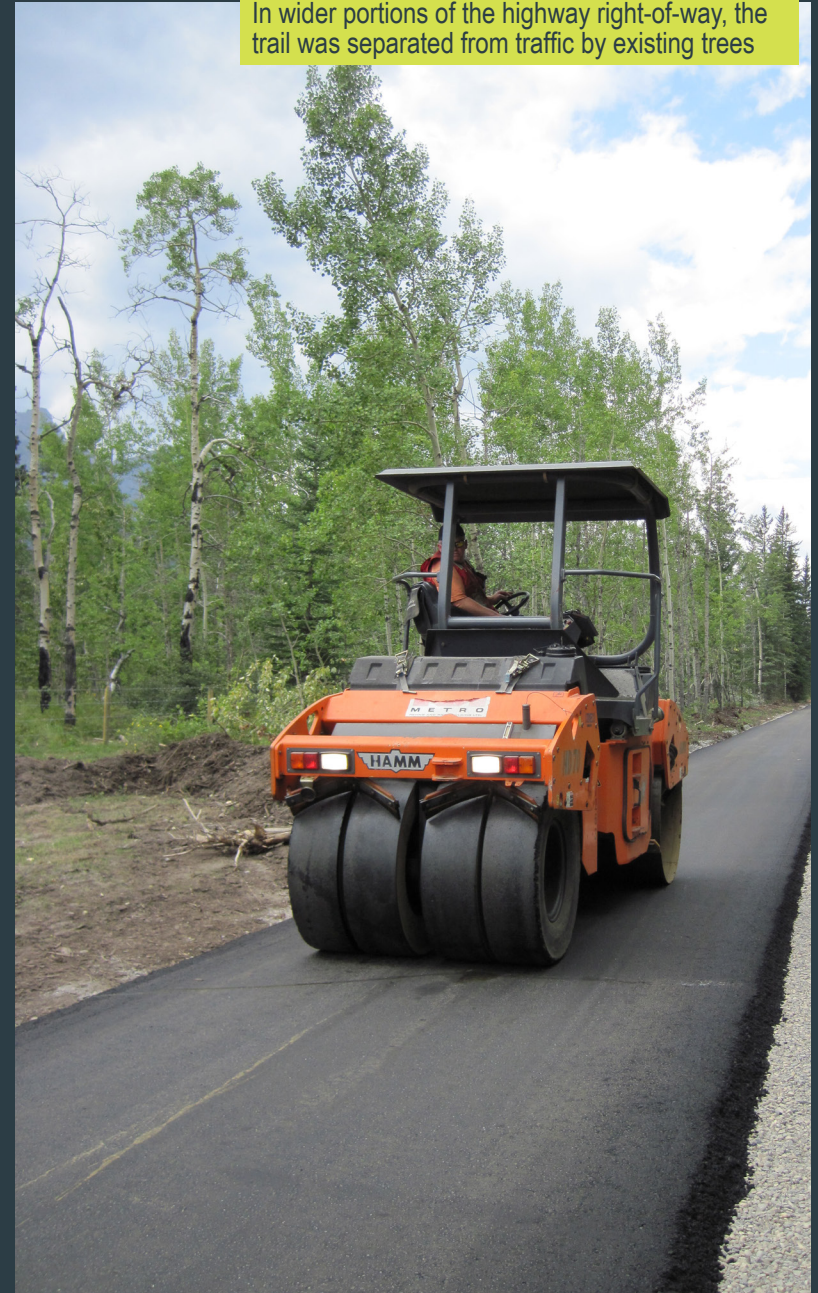
Asphalt paving was completed in one lift for improved efficiency
