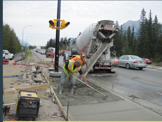
Construction of trailhead bus stop plaza using synthetic fiber-reinforced concrete
