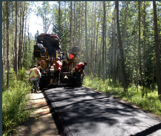
Asphalt paving was completed in one lift for improved efficiency
