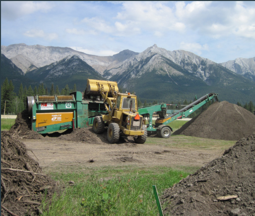
Screening local topsoil on site for rehabilitation work
