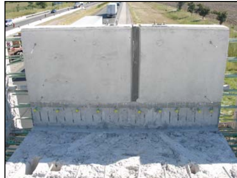
(b) Prefabricated Link Slab Panel showing Expansion Joint in Parapet Wall
