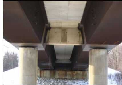
(b) Completed Concrete Diaphragm
