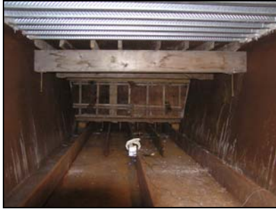
(a) Formwork inside Box Girder
