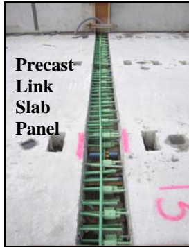
(a) Reinforcement Continuity Provided by Mechanical Couplers
