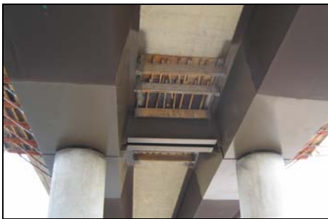
(a) Formwork at Soffit of Link Slab
