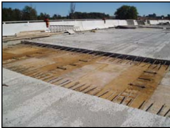
Figure 11: Removal of Strip of Deck Slab at Pier
