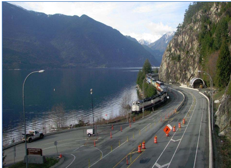
Figure 8: 3 rd lane on rail bed at Porteau closed temporarily to allow passage of train
