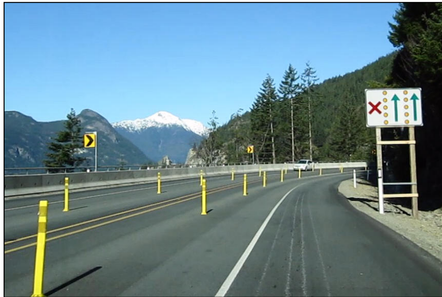
Figure 6: Fixed delineator marker posts and directional signage for lane counterflows
