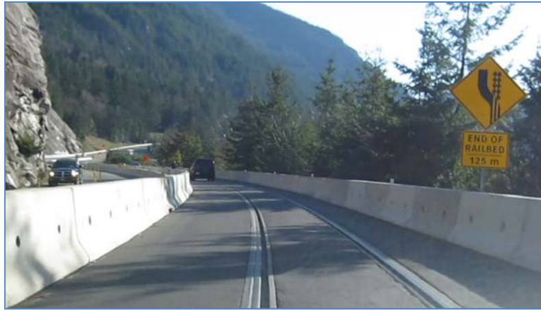
Figure 7: 3 rd lane on CN rail bed at Porteau to provide additional southbound capacity
