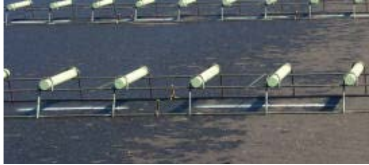
Figure 1: Dowel Basket Assembly
