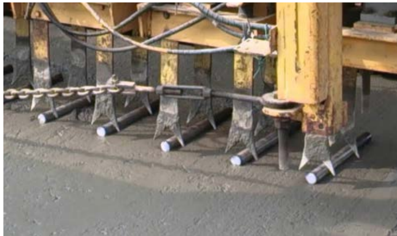
Figure 2: Dowel Bar Inserter on Slipform Paver
