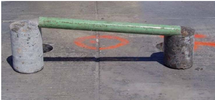
Figure 4: Cored Dowel Bar Ends with Representative Bar to Show 3D Bar Alignment (Yu 2005)
