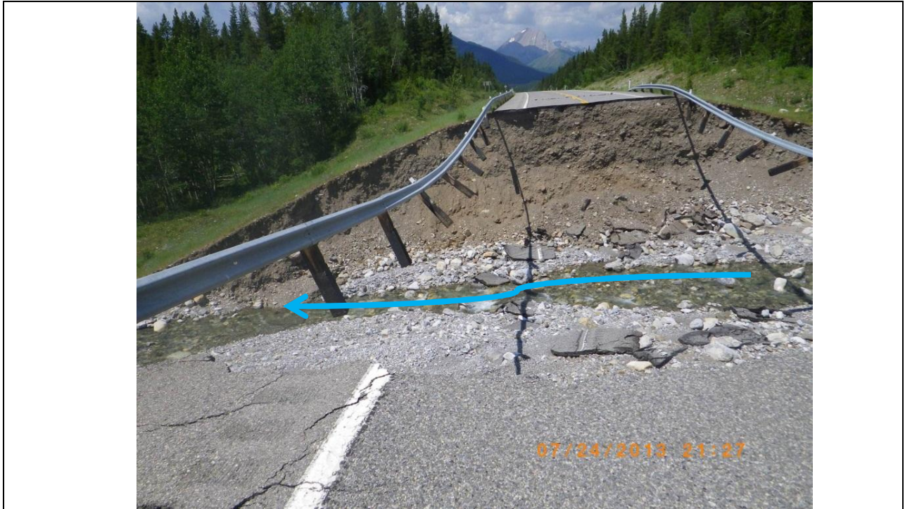
Photoplate 5 - Site 133 Lineham Creek site facing north; Facing downstream
