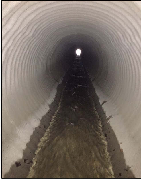
Figure 10 – Completed Geopolymer Mortar Lining
