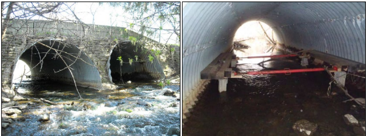
Figures 11 – Culverts prior to Rehabilitation
