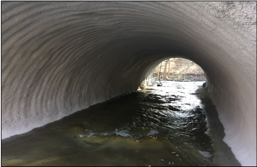
Figure 13 – Completed Culvert Lining
