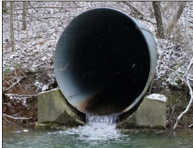
Figure 8 – Existing Culvert at SR 446
