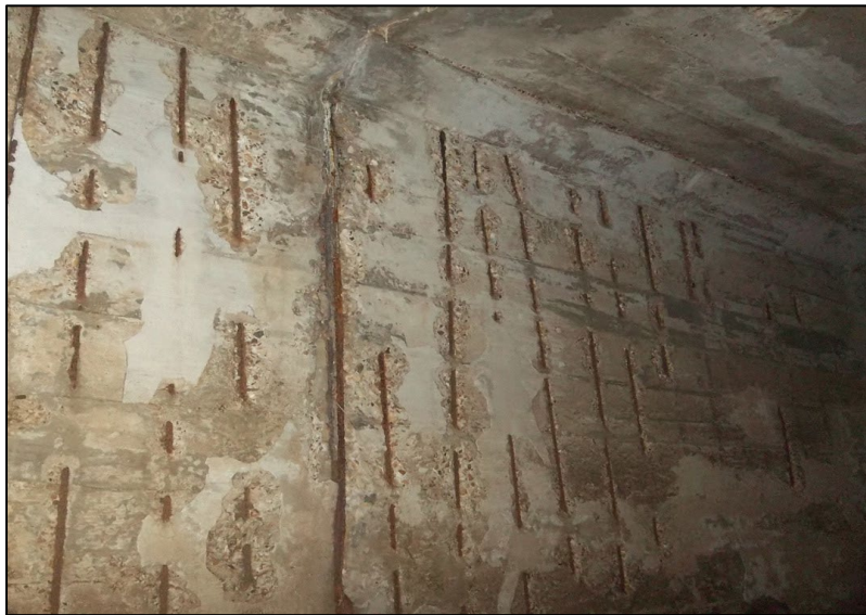
Figure 15 – Cleaned Wall Section Ready for Lining
