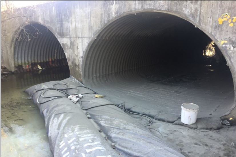
Figure 12 – Flow in the Stream Channel was Maintained by Flow Diversion
