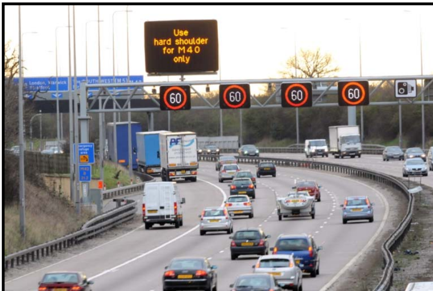
Figure 3 – Once the hard shoulder is open, the speed limit is set to 60 mph (the default speed limit on UK motorways being 70 mph) or to a lower limit should conditions warrant
