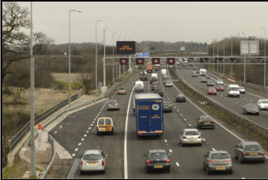
Figure 1 - MM-DHS with Emergency Refuge Area
