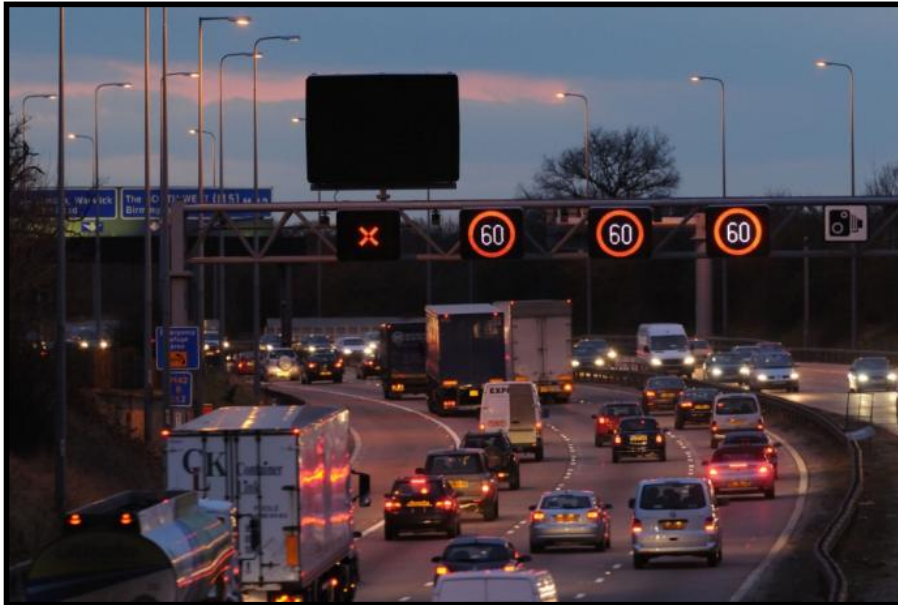
Figure 2- During the conditioning phase, the speed limit on open lanes is set to 60 mph and a “Red X” is shown over the hard shoulder to reinforce the fact that it remains closed to traffic.
