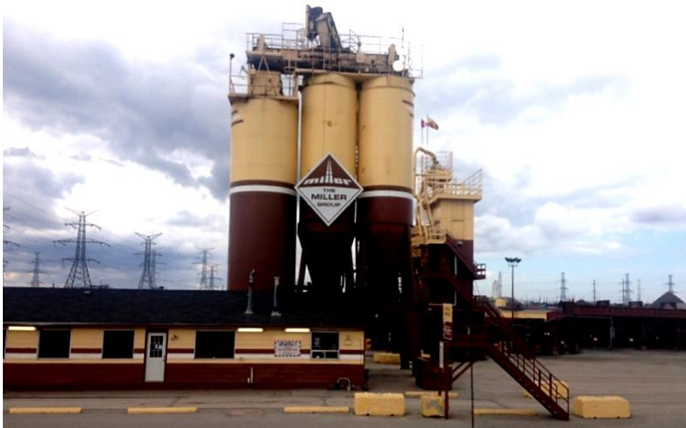
FIGURE 1 Miller Group batch plant
