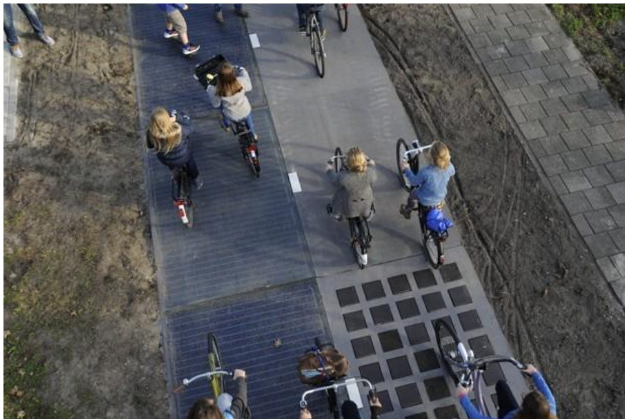
Figure 7: SolaRoad, the world's first solar bike path, in Normandy
