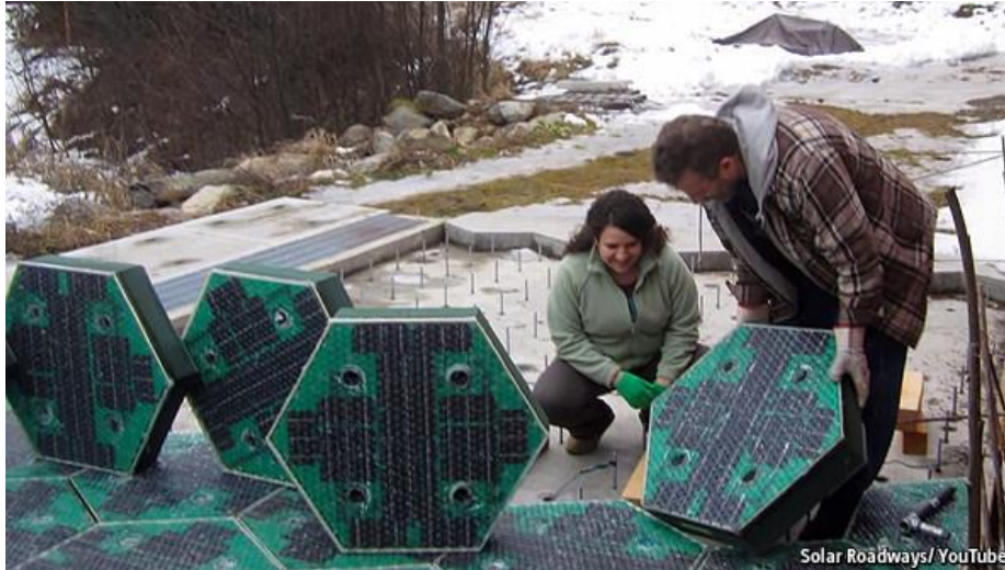
Figure 8: Solar Roadways® has developed interlocking hexagonal panels
