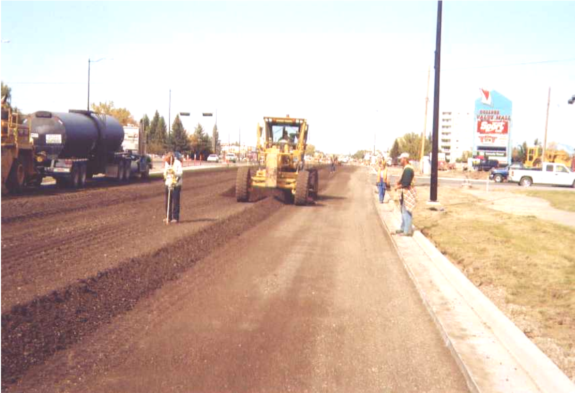
Figure 4: FDR Grading Operations
