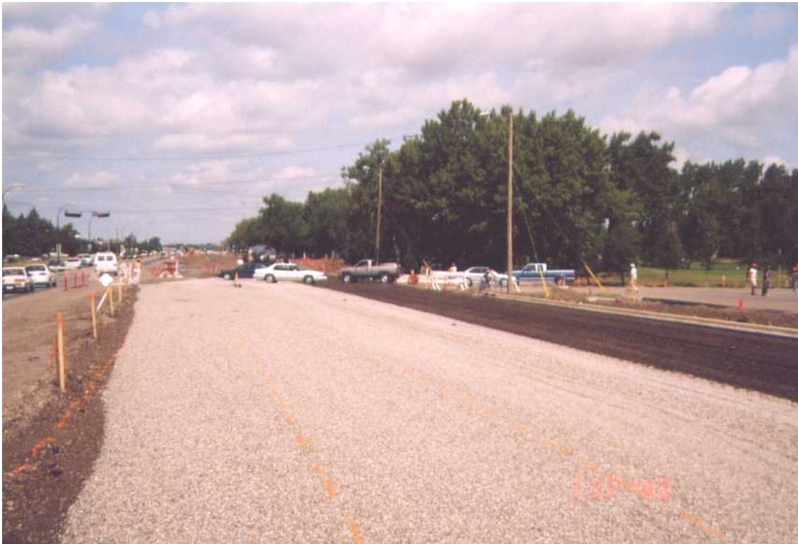
Figure 2: Traffic Accommodation during FDR Stabilization
