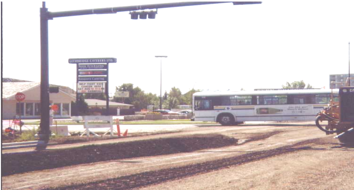
Figure 3: Continuous Transit Bus Service during Construction
