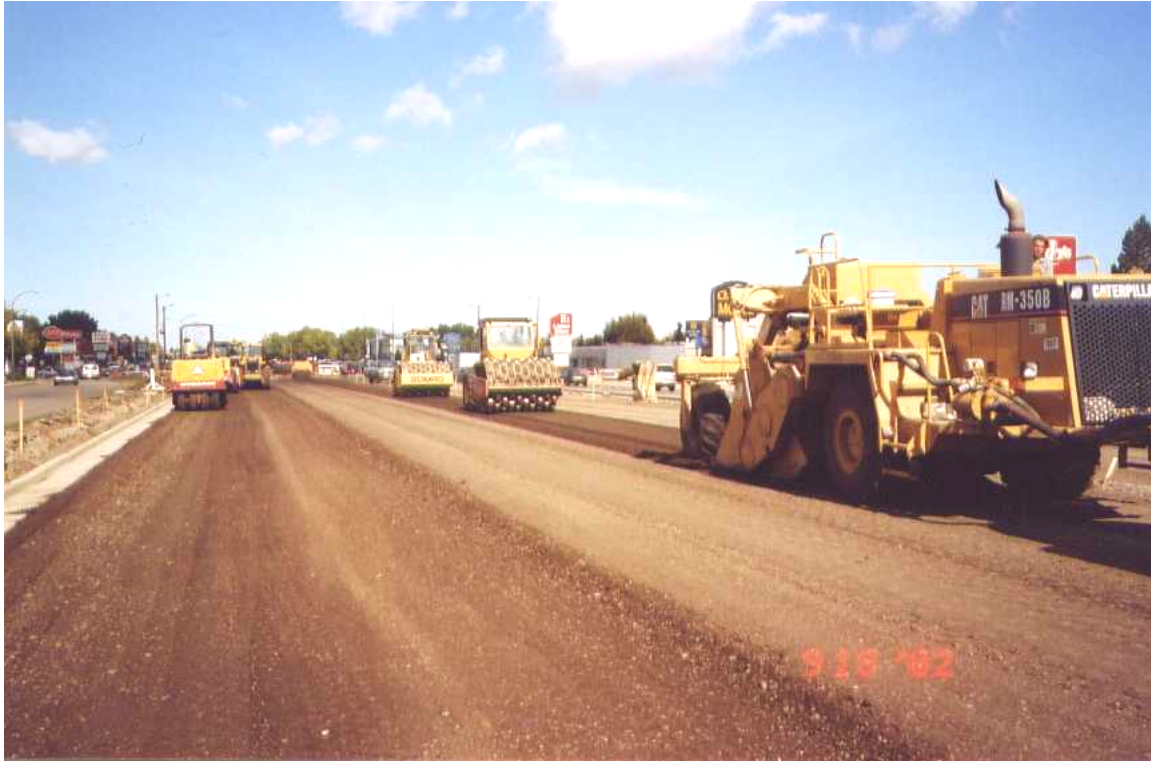
Figure 5: FDR Compaction Operations
