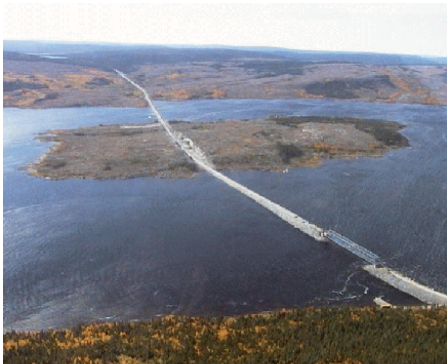
FIGURE 6 Aerial View of Alexis Bridge and Causeway
