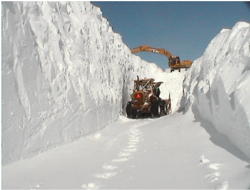
FIGURE 8 Winter Maintenance on Trans Labrador Highway
