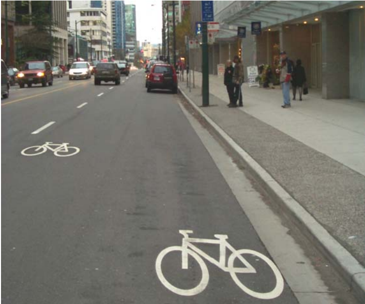
Figure 14: Side-by-Side Application with Part Time Parking, on Pender St, Vancouver BC
