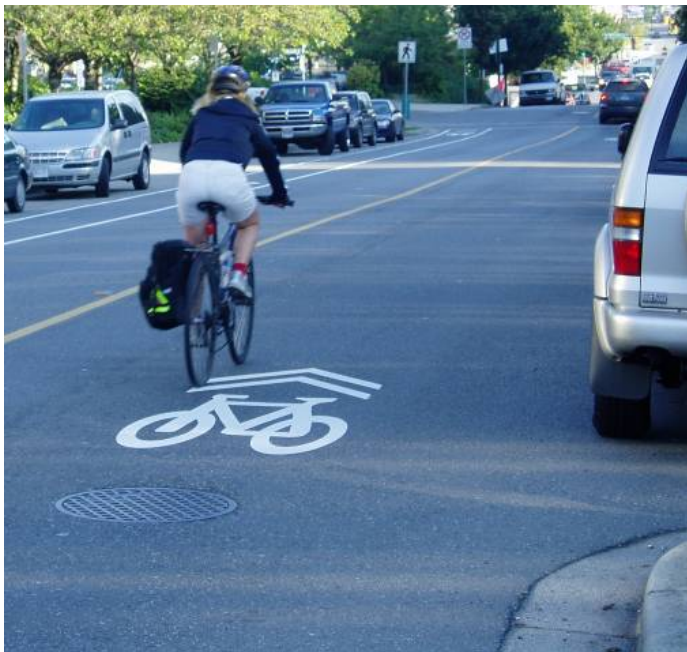
Figure 13: Single File Sharrow Application on Yukon St, Vancouver BC
