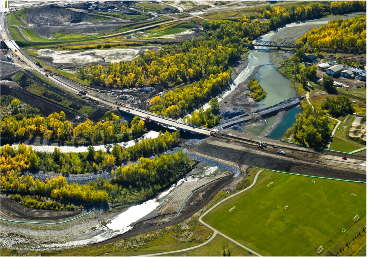
McAlpine (32 Street) Crossing - Sheep River Re-Alignment Project
