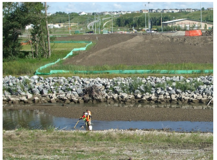
Fish Salvage and Relocation
