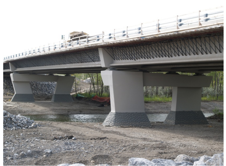
Sheep River Bridge
