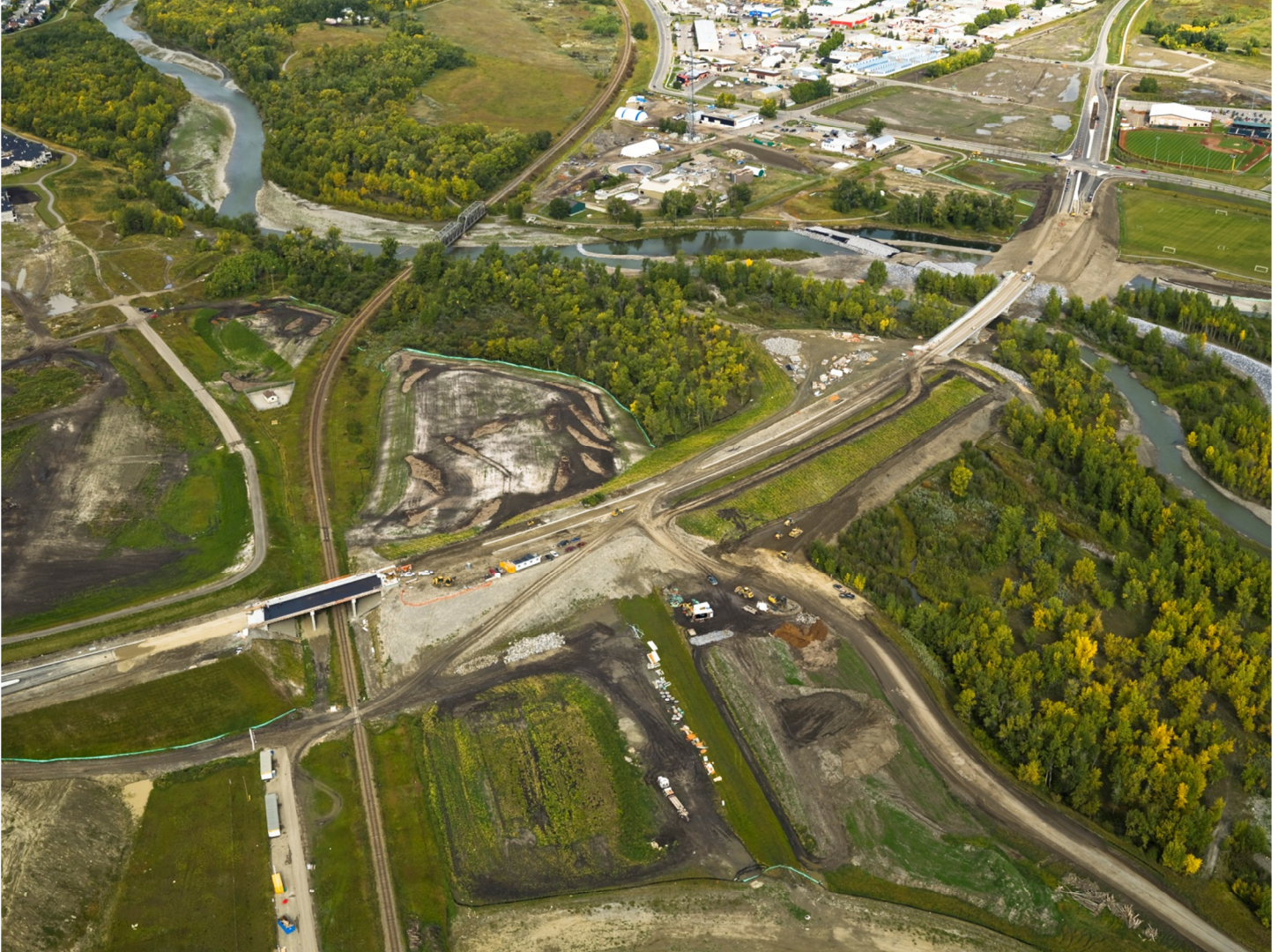
32 Street Crossing - Sheep River Re-Alignment Project
