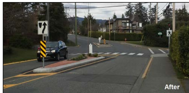
Resthaven Drive at Ardwell Avenue (Sidney, BC): Photos show pedestrian crossing improvements (median island and side-mount pedestrian flashers) made in 2014, using a $6,000 contribution from the Road Improvement Program.
