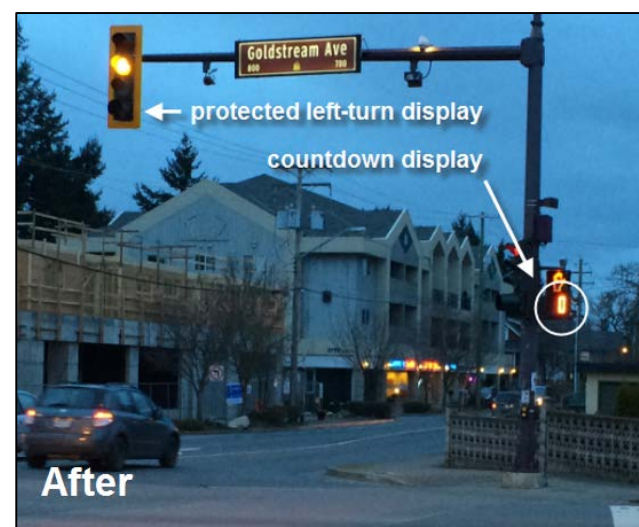
Intersection of Goldstream Avenue and Peatt Road (Langford, BC): Photos show signal upgrades (protected left turns and pedestrian countdown heads) made in 2014, using a $17,000 contribution from the Road Improvement Program.
