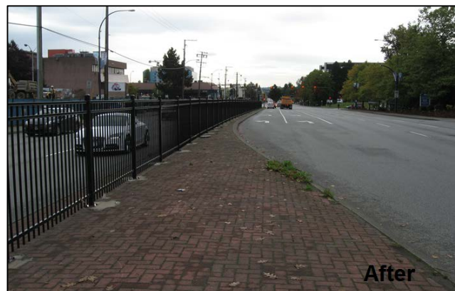
King George Boulevard, 98B Ave to Fraser Hwy (Surrey, BC): Photos show corridor improvements (installation of median fence to reduce jaywalking) made in 2014, using a $25,000 contribution from the Road Improvement Program.
