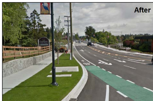
Craigflower Bridge (View Royal, BC): Photos show corridor improvements (added vehicle and cycling lanes, improved pedestrian facility, improved lighting) made in 2013/14, using a $250,000 contribution from the Road Improvement Program.
