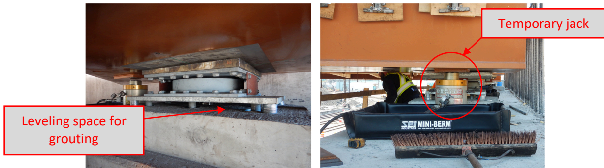
Figure 19: Temporary jacks and bearing assembly
