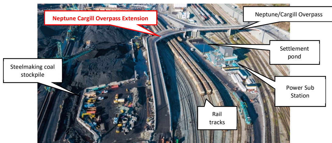
Figure 5: Overview of Site, looking west (after completion of overpass construction)
