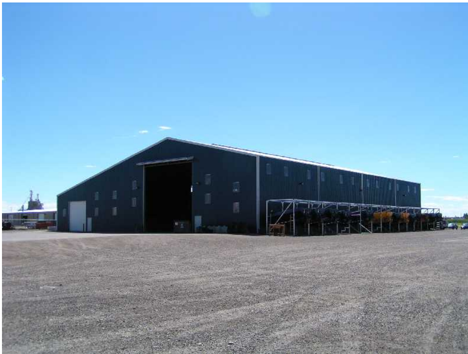
Figure 2: Steel Sand/Salt Storage Structure (Lethbridge)
