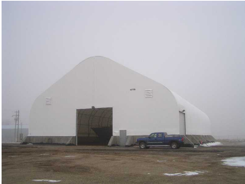
Figure 3: Fabric Sand/Salt Storage Structure (Nanton)
