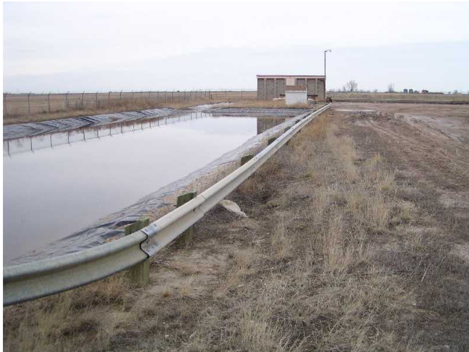
Figure 4: Retention Pond (Taber)
