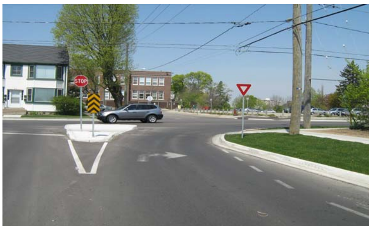
Fig. 14, example of an urban smart channel used elsewhere in the City of Waterloo
