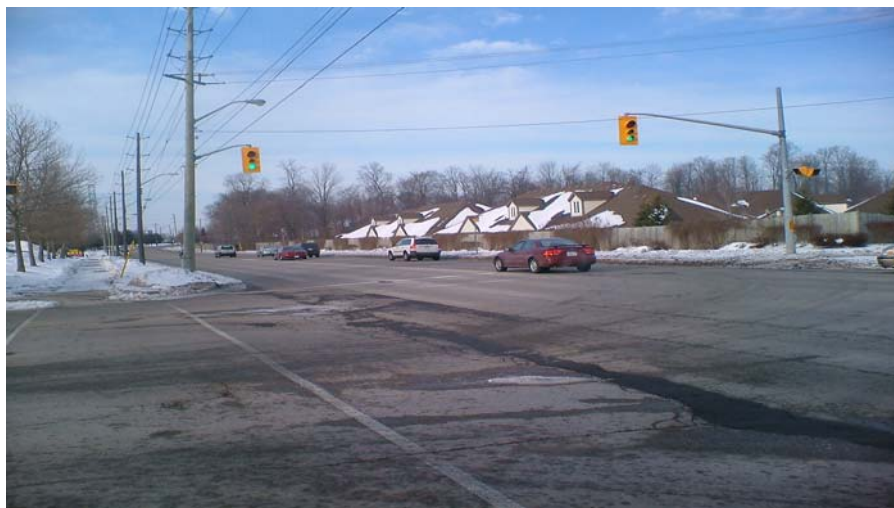
Fig.10, Davenport Road is wide and straight with sight distances in excess of those required onto intersection. Identified as third worst collision intersection in city in 2008
