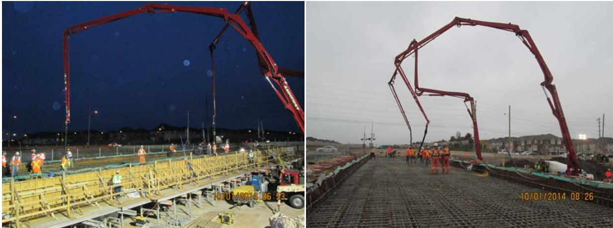
Photo 2: Continuous Concrete Deck Pour
