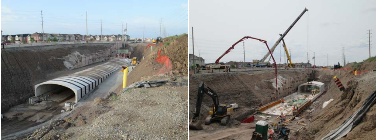
Photo 3: Installation of precast detention tank
