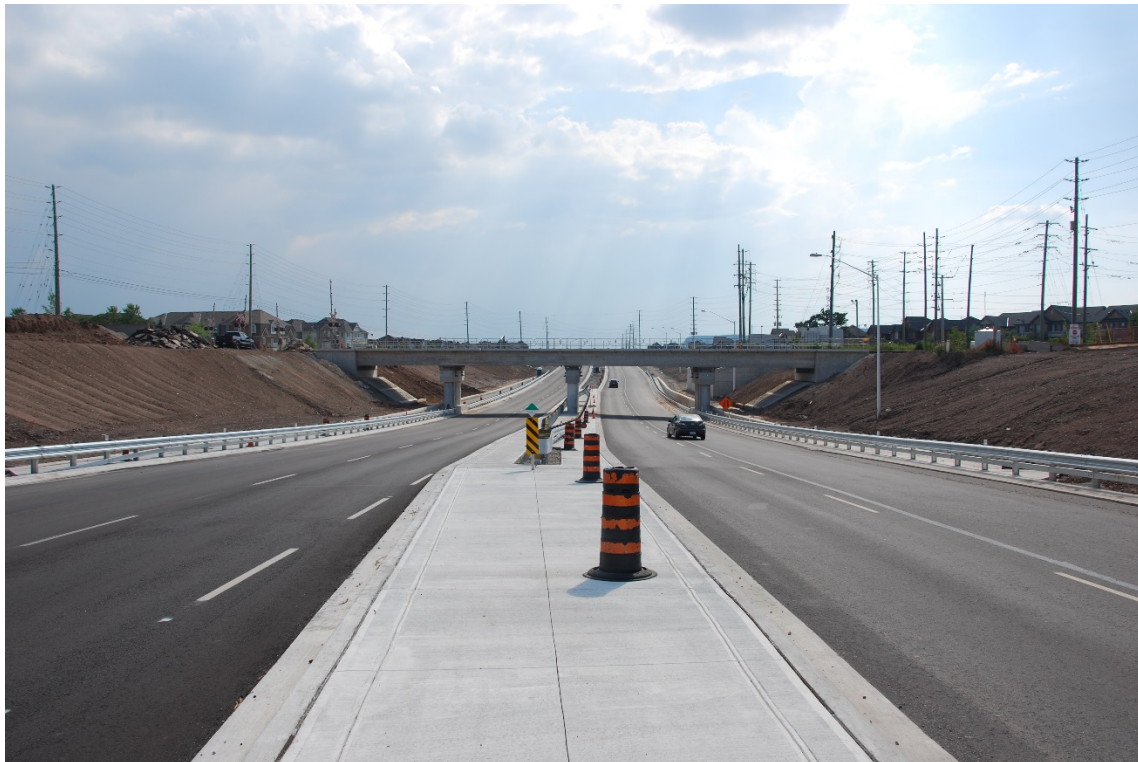
Photo 1: Grade Separation looking westbound
