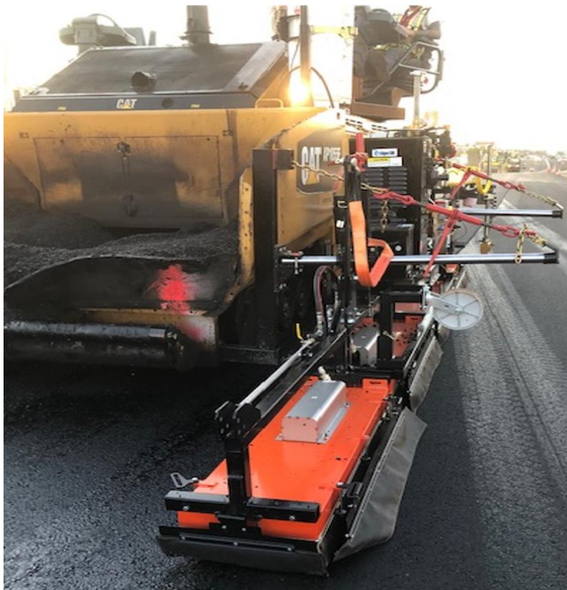
Figure 9 Joint Heater Attached to the Paver on City of Calgary Projects
