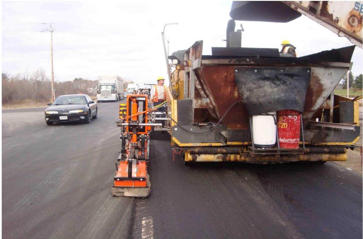
Figure 8 HDE Infrared Joint Heater Attached to the Paver [10]
