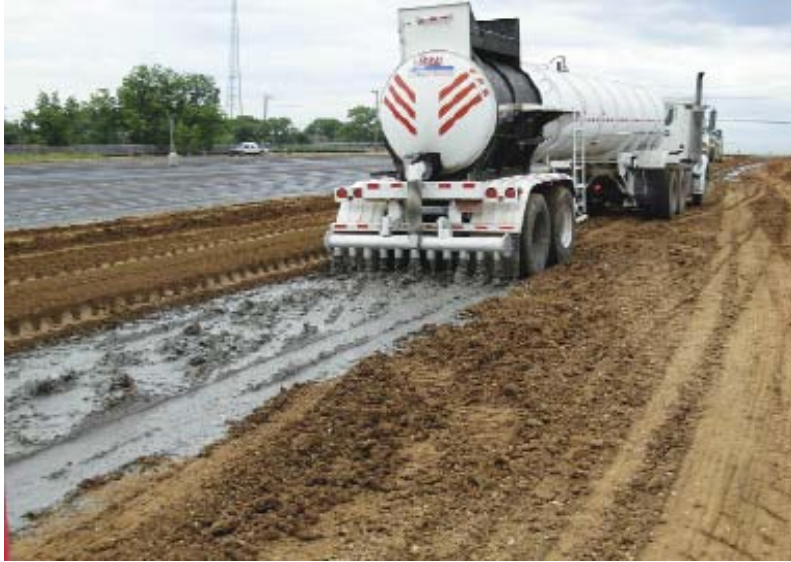
Figure 7 - Distributing cement in slurry form from a distributor truck.
