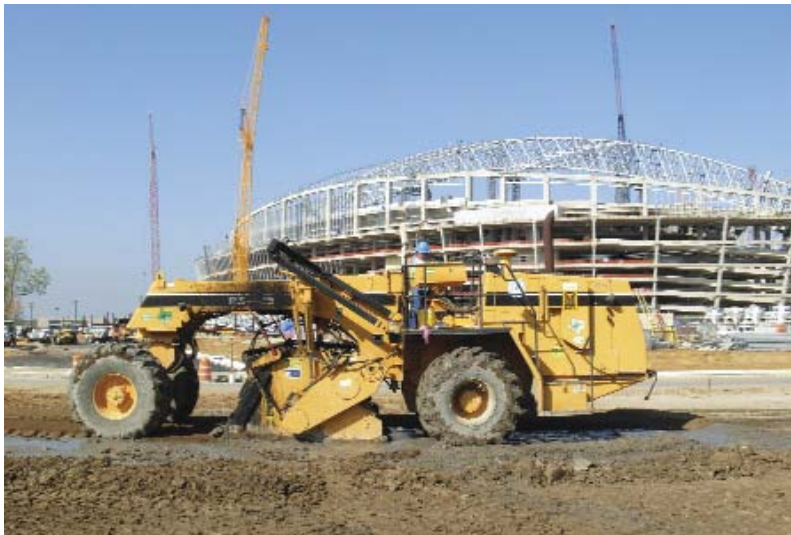
Figure 1 – In-place mixing for modification of clay soils at the Dallas Cowboys Stadium.
