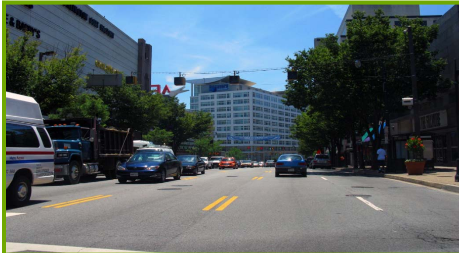
Figure 4 – Lane Striping - Coleville Road, MD
