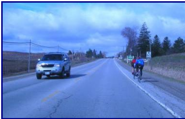
Figure 8 – Example of a Paved Shoulder Bikeway in York Region (MMM Group Ltd.)
