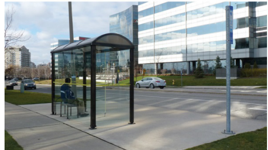
Figure 1: Public Transit Stop in an Employment Area
