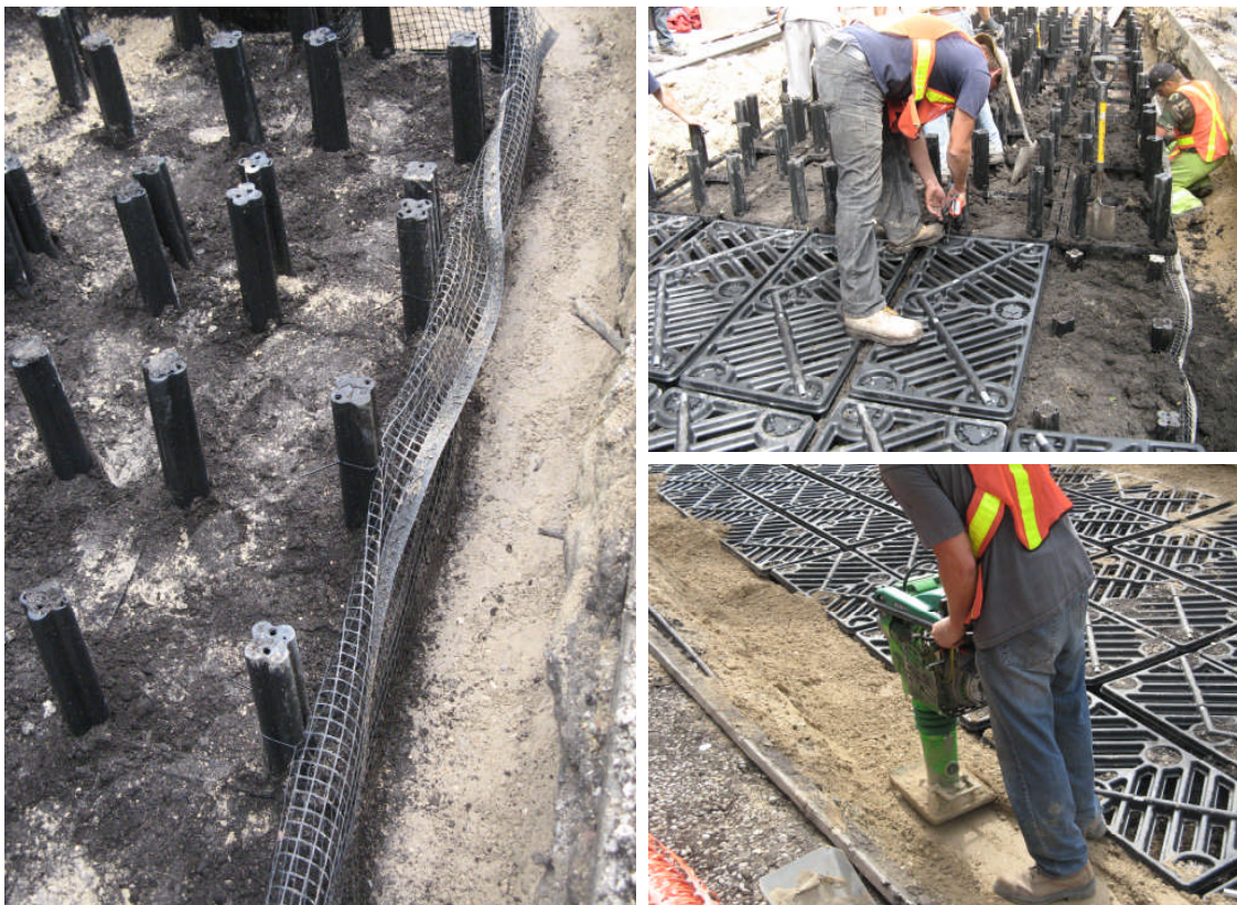
Figure 4 – Structural Cells Being Wrapped, Filled and Covered in Winnipeg
