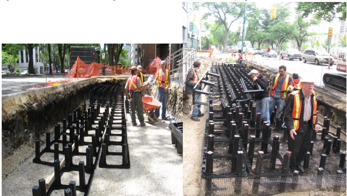
Figure 2 – Structural Cells Being Stacked on Each Other in Winnipeg
