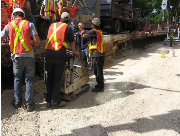
Figure 3 – Typical Construction Methods Used (bedding compaction shown here)
