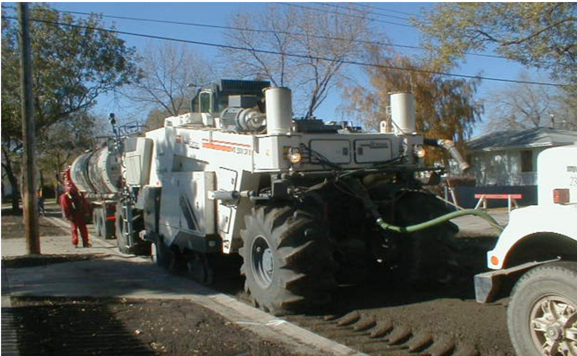
Figure 6 Roadway Reconstruction, Full Depth Reclamation
