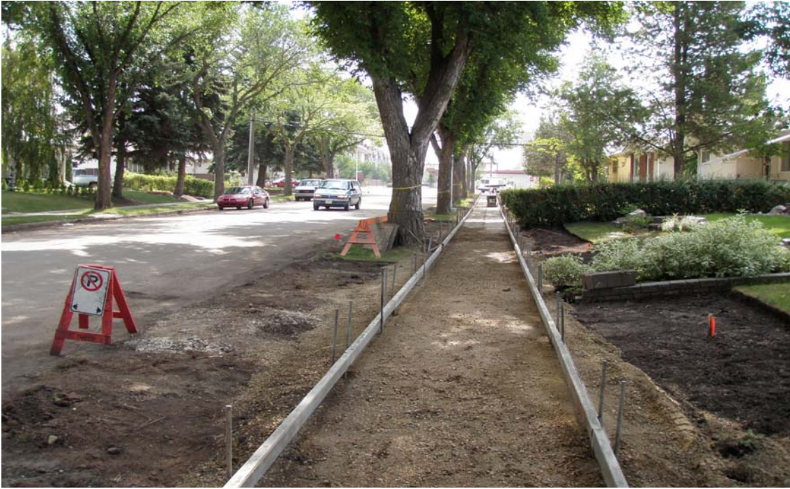
Figure 3 Hand Concrete Sidewalk Replacement
