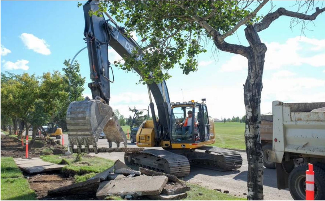
Figure 2 Concrete Removal
