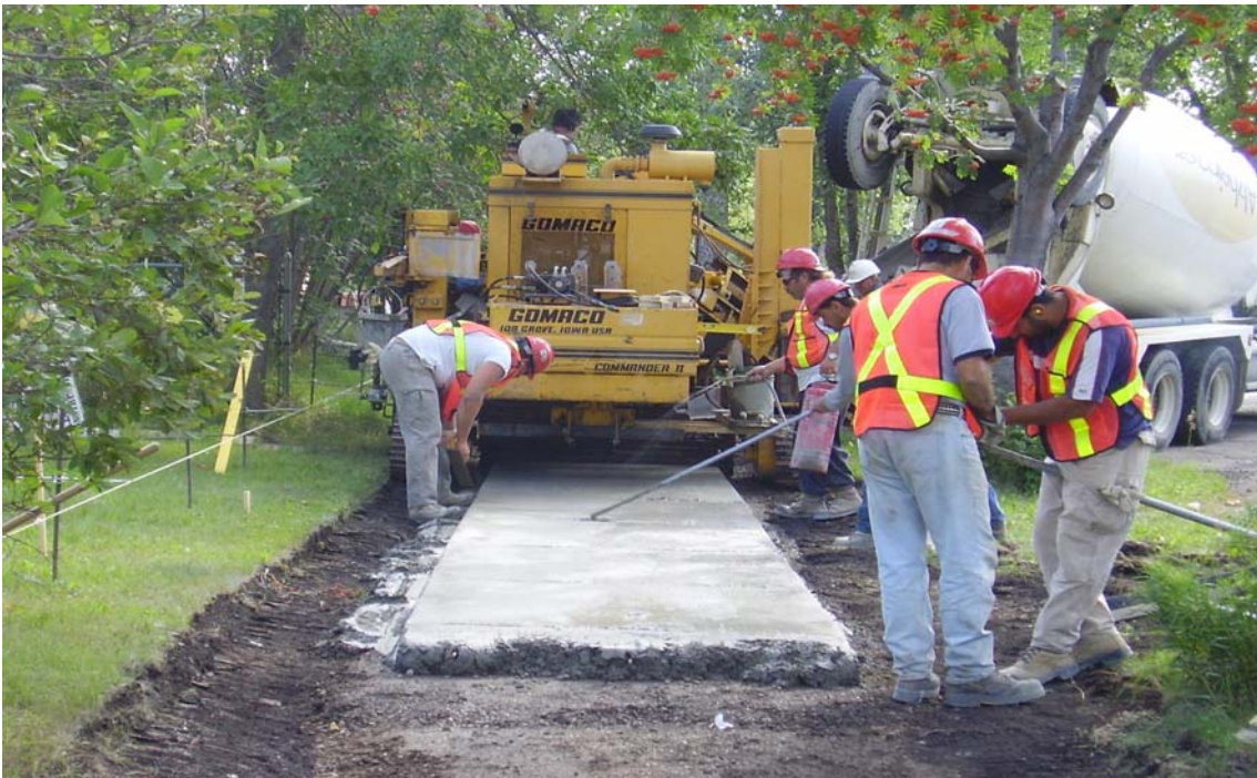
Figure 4 Machine Concrete Sidewalk Replacement
