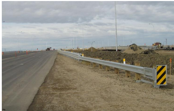
FIGURE 6: EAGRT installed with 10:1 flare
