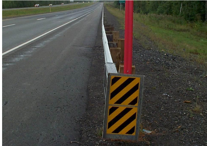
FIGURE 5: EAGRT installed with 100:1 flare
