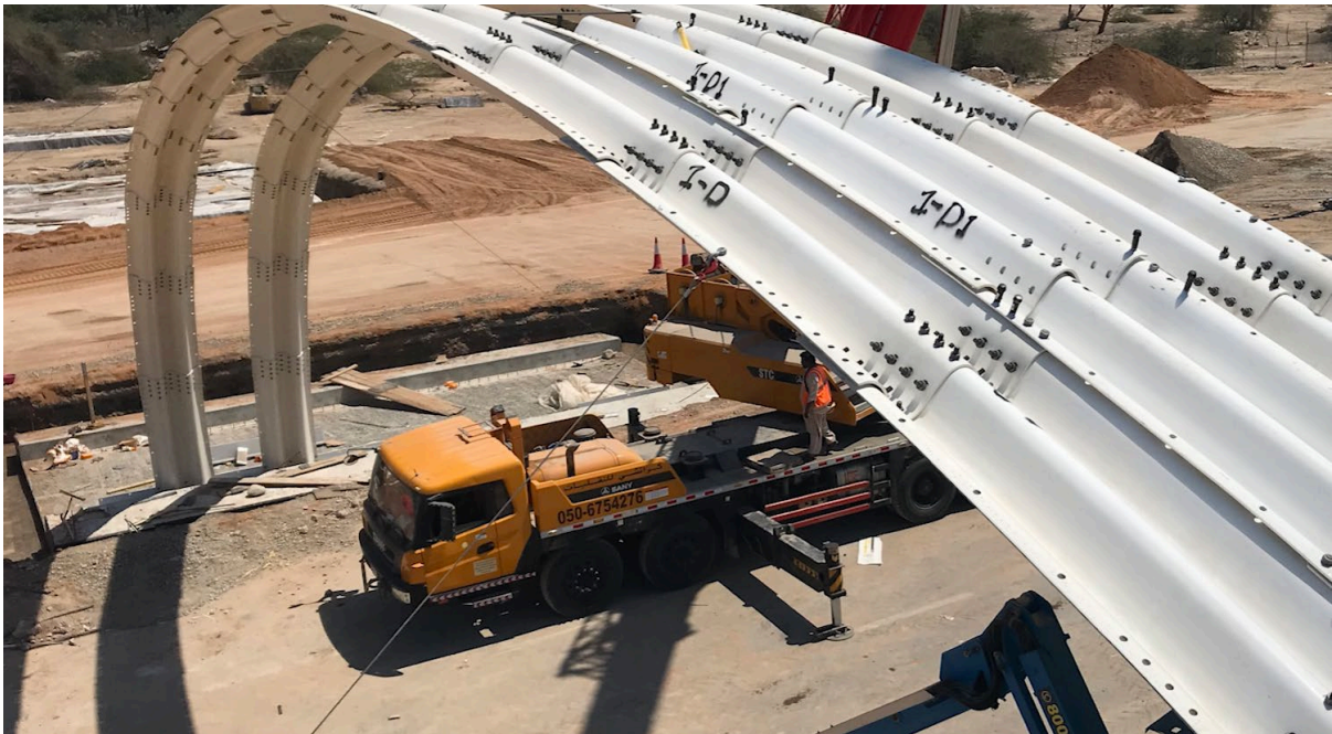
Figure 8: Photo of erection of first three rings
