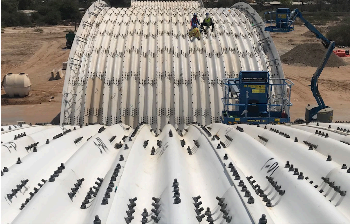
Figure 9. Photo for structure assembly near completion
