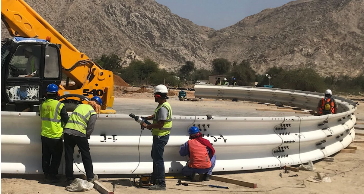
Figure 7 Photo for first ring assembly.
