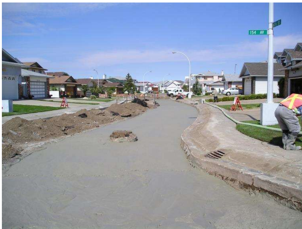
Figure 6 - Cellular concrete after placement along 67A Street NW, Edmonton, Alberta
