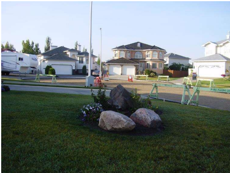
Figure 11 - Completed Granular Layer on the Lightweight Concrete Layer on 62 Street NW, Edmonton, Alberta
