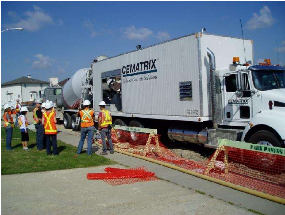
Figure 5 - Lightweight Cellular Concrete Wet Mix Equipment
