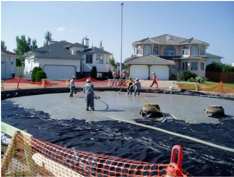
Figure 9 - Placement of Lightweight Cellular Concrete on 62 Street NW, Edmonton, Alberta
