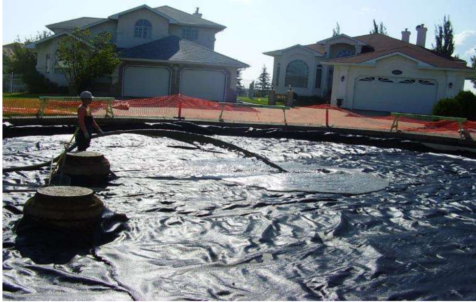
Figure 8 - Placement of Lightweight Cellular Concrete on 62 Street NW, Edmonton, Alberta
