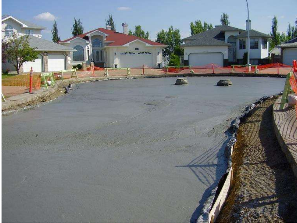
Figure 10 - Completed Lightweight Cellular Concrete on 62 Street NW, Edmonton, Alberta
