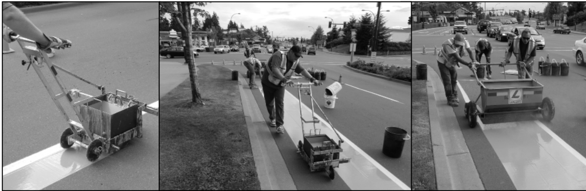
Photo I: First steps of application process of Lafrentz SRM MMA and bauxite
