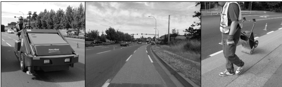
Photo II: Second steps removing excess bauxite and sealing surface with MMA resin
