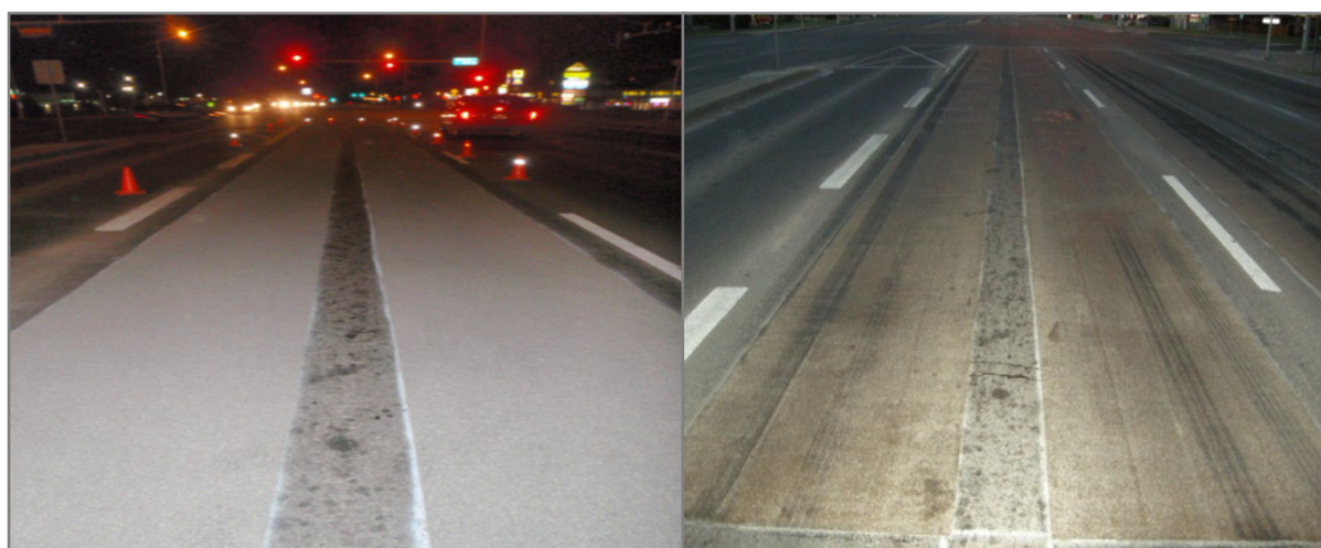
Photo III: Post Installation Photo
