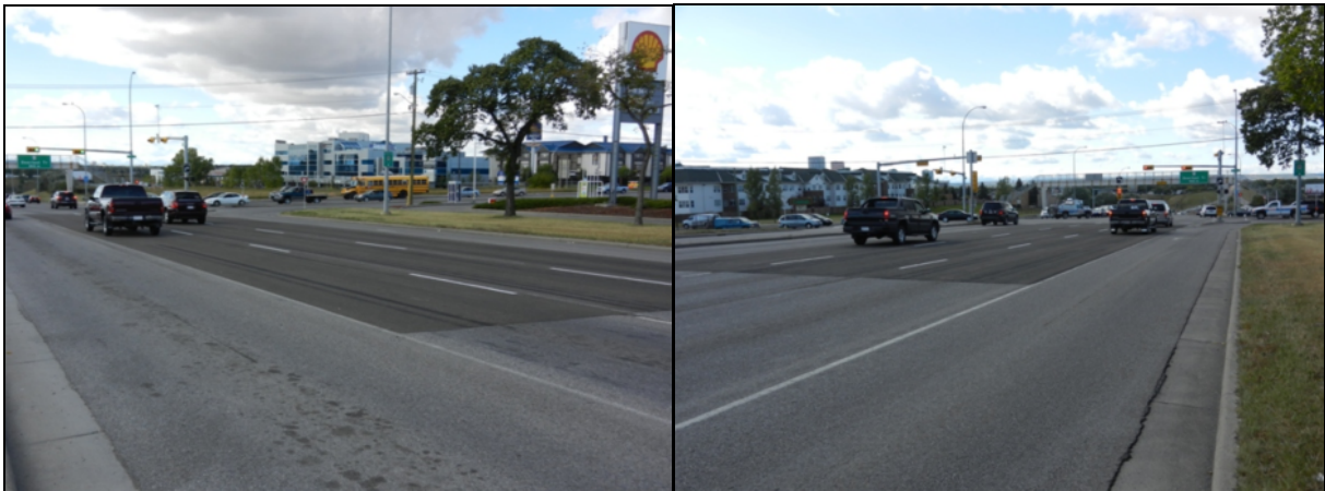
Photo V: Solid Laneway Application of SRM
